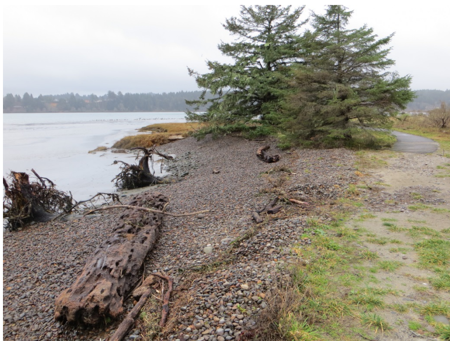
Figure 41. A cobble berm or dynamic revetment, constructed adjacent to the Hatfield Marine Science Center in Yaquina Bay, has successfully stopped erosion of the backshore. (Photo credit: J. Allan, DOGAMI, 2016)
