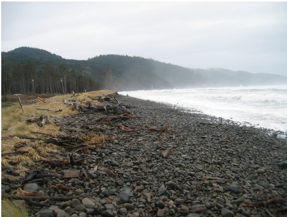
Figure 2-23. Dynamic revetment “cobble beach” constructed at Cape Lookout State Park. The cobble beach is backed by an artificial dune, which periodically is overtopped during major storms (photo: J. Allan, DOGAMI, 2008).
