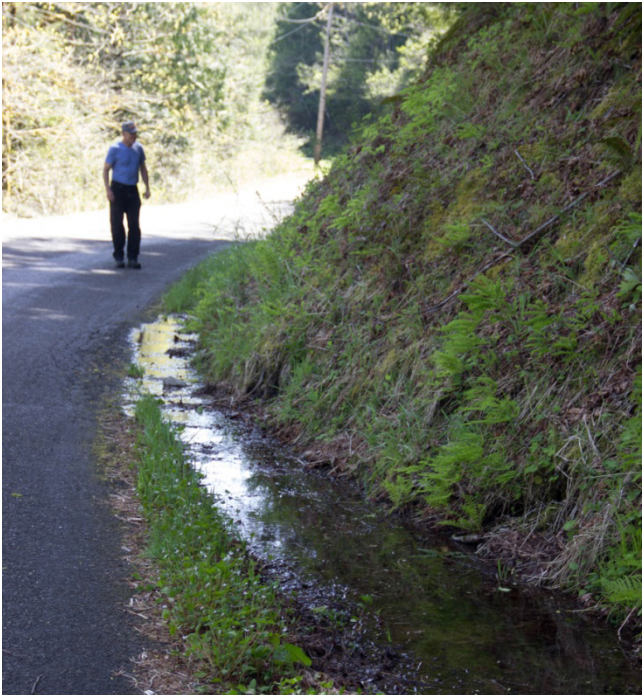
Figure 21. Photo of the toe of an historic/active landslide along NF road 10. Photo location is at the green star in Figure 20. The toe appears to be over-steepened through grading. At the time, the photo was taken water was pouring out of the slope and filling the ditch. (Photo credit: K. A. Mickelson)
