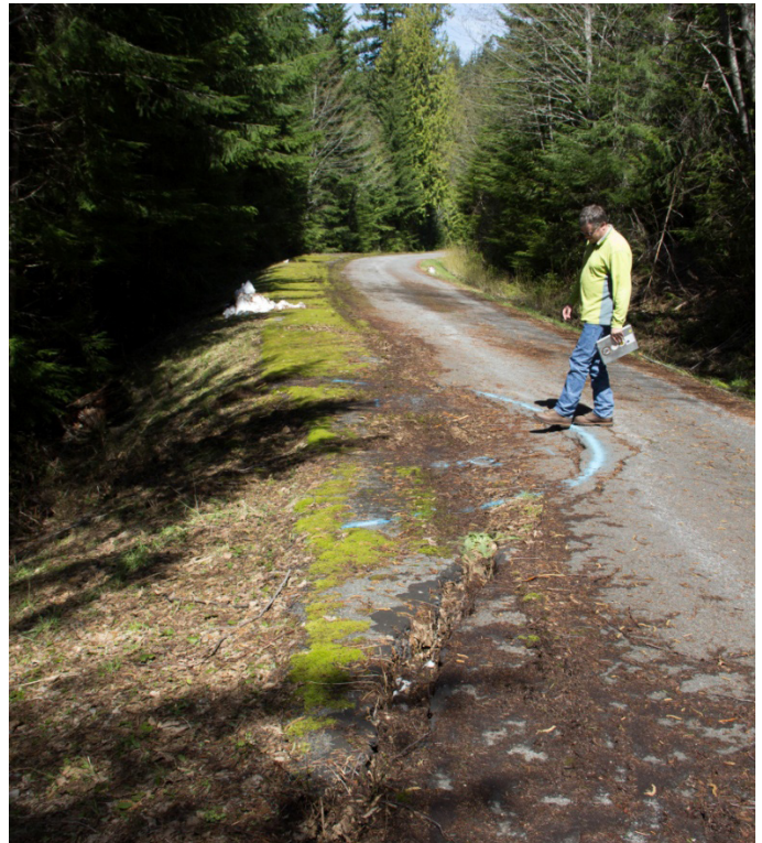
Figure 18. Road fill embankment failure along NF road 10 in southeastern Bull Run Watershed. (Photo credit: K. A. Mickelson)
