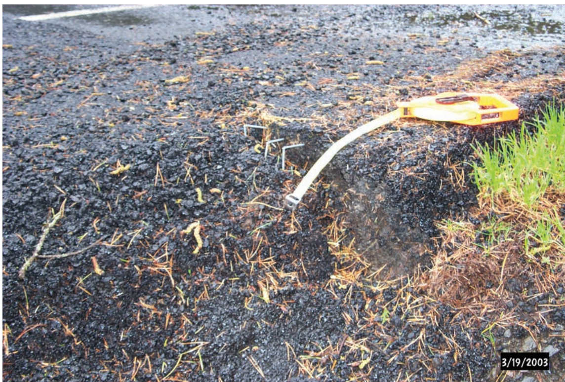
Figure G14. Marker nail site JC-22 looking southeast on west side of U.S. Highway 101. Scarp is asphalt and gravel.
