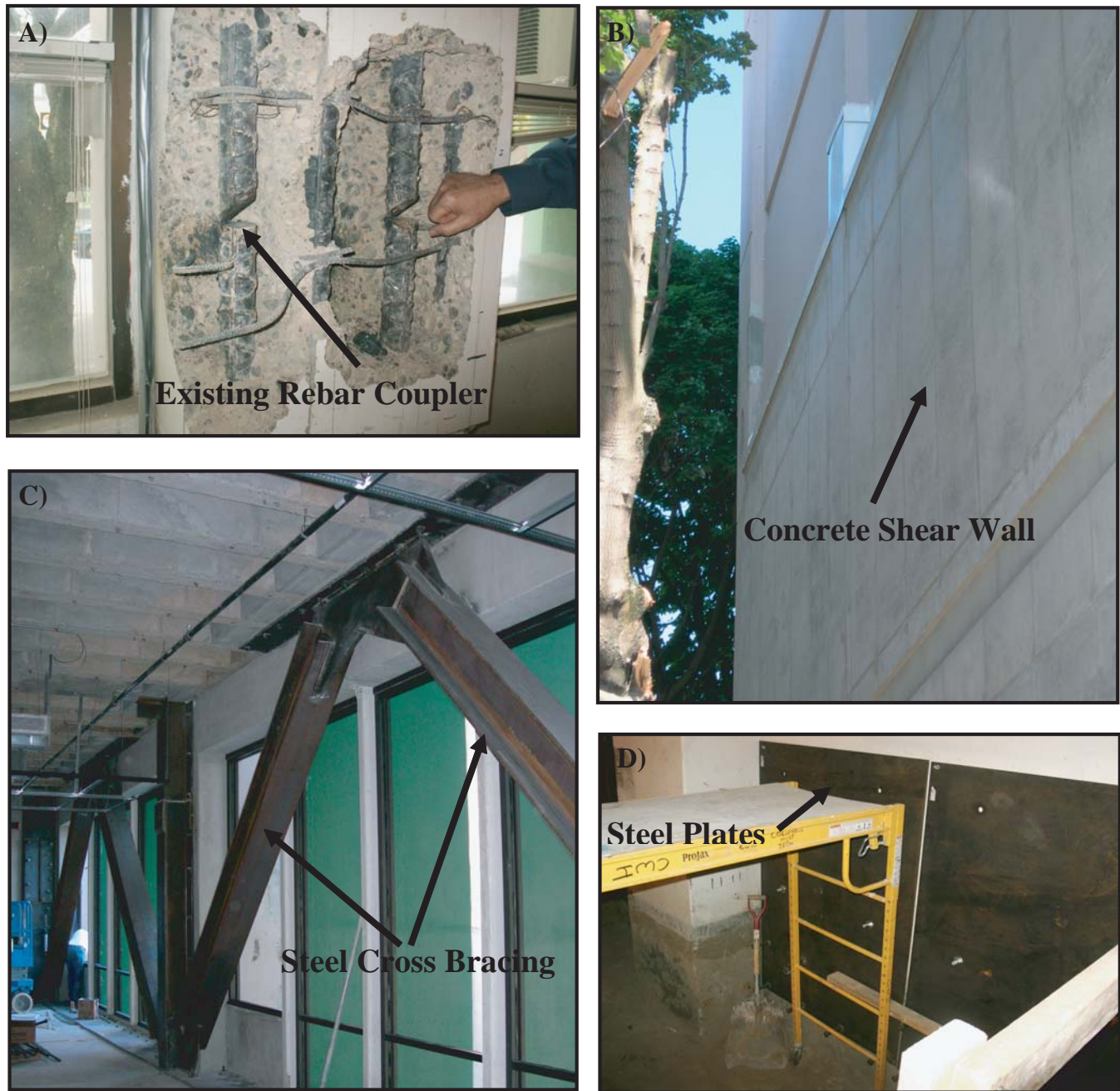
Figure 5. Solutions recommended by structural engineers for seismic improvement: (A) existing rebar joint, which was mitigated by welding rebar together, (B) new concrete shear wall on the south side of the building, (C) new steel cross bracing, and (D) steel plate installation in progress.
