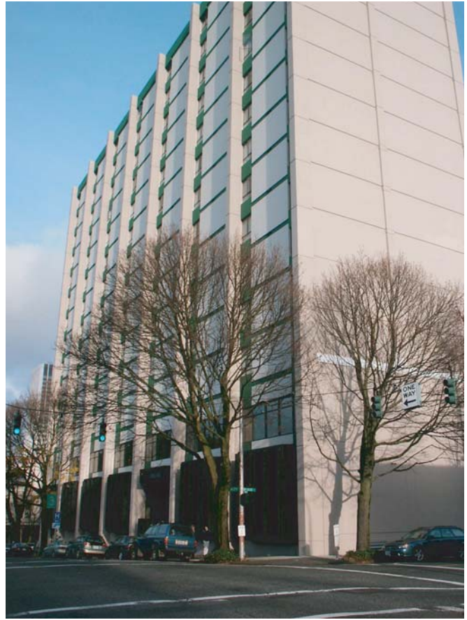
Figure 1. Ondine Residence Hall, Portland State University. This view from the southwest shows the lower, soft stories that are vulnerable to collapse prior to mitigation.
