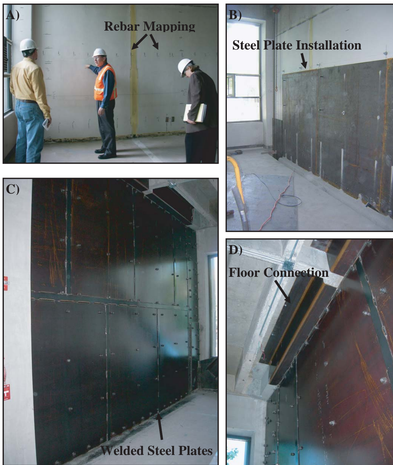
Figure 11. Construction process for steel plates: (A) rebar mapping, (B) installation in progress, (C) completed wall with sheets welded together, and (D) plate connected floor to floor.
