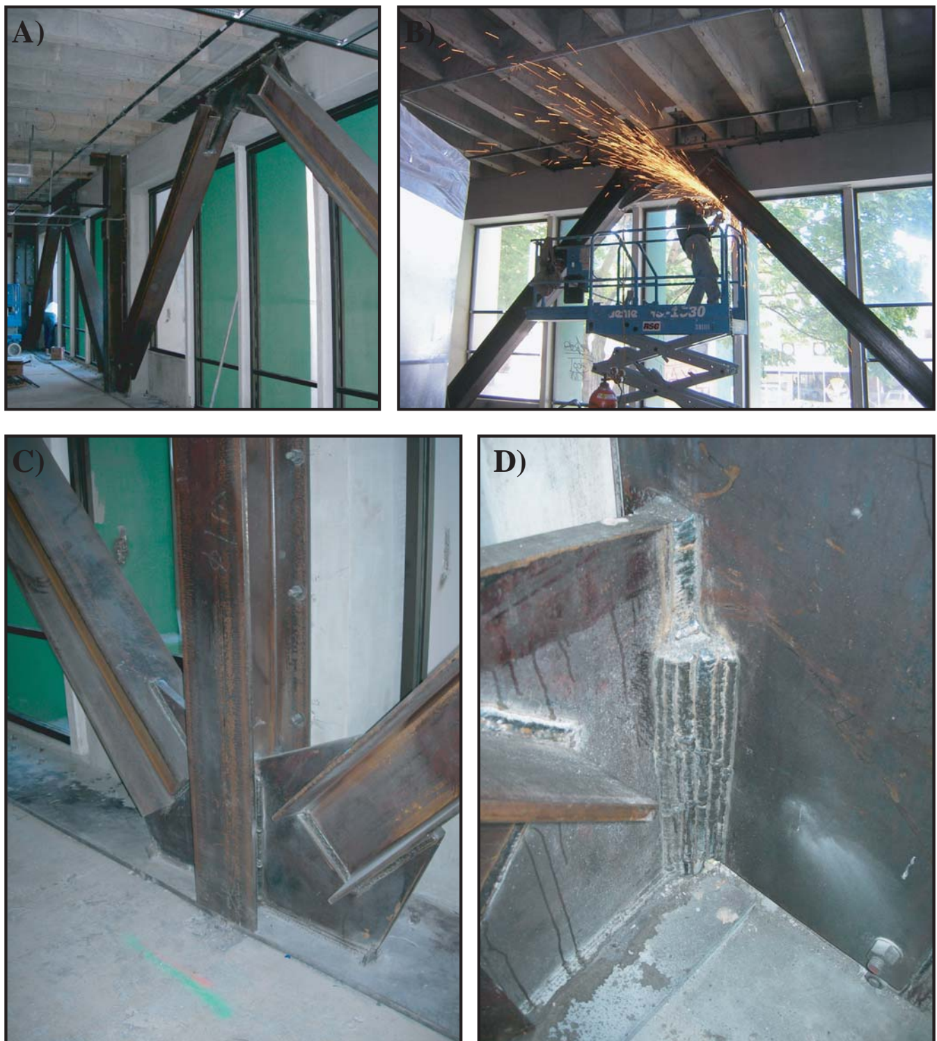
Figure 12. Construction of cross-bracing on first and second stories along west elevation: (A) Installed cross-bracing, (B) cross-bracing installation in progress, (C) close up of welded plate at floor level, and (D) close-up of weld used to connect new cross-bracing to steel plates.
