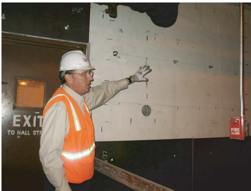
Figure 7. Map of existing rebar to determine locations for drill hole anchors needed for steel plate mitigation.
