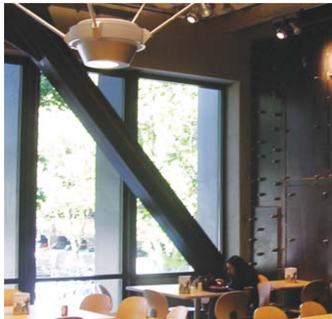
Figure 13. New structural cross-bracing and a wall of steel plates, burnished for aesthetic reasons, are permanently visible in Ondine Hall cafeteria.
