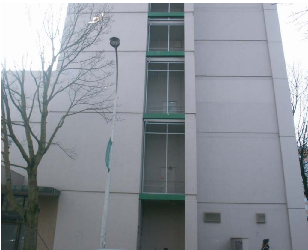
Figure 6. Obstacles such as the exterior stairwell prevented use of additional exterior concrete shear walls.
