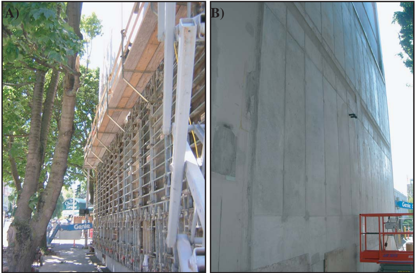
Figure 10. Construction of concrete shear wall along south side of Ondine Hall: (A) preparing new portion of concrete shear wall, and (B) completed shear wall.
