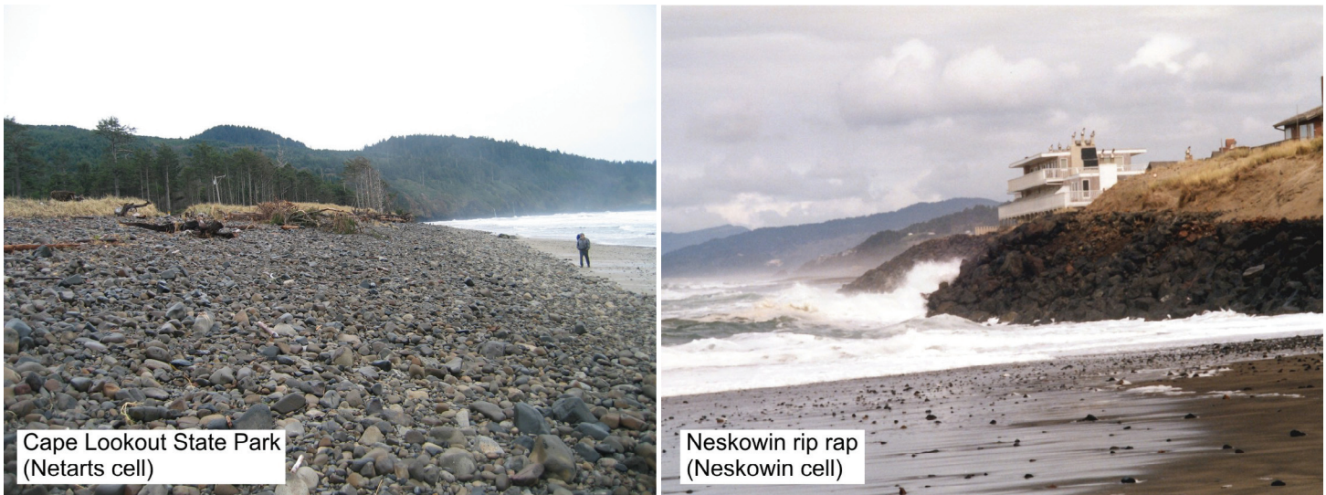
Figure 16. Comparison of a dynamic revetment constructed at Cape Lookout State Park (left) versus a conventional riprap revetment constructed at Neskowin (right).
