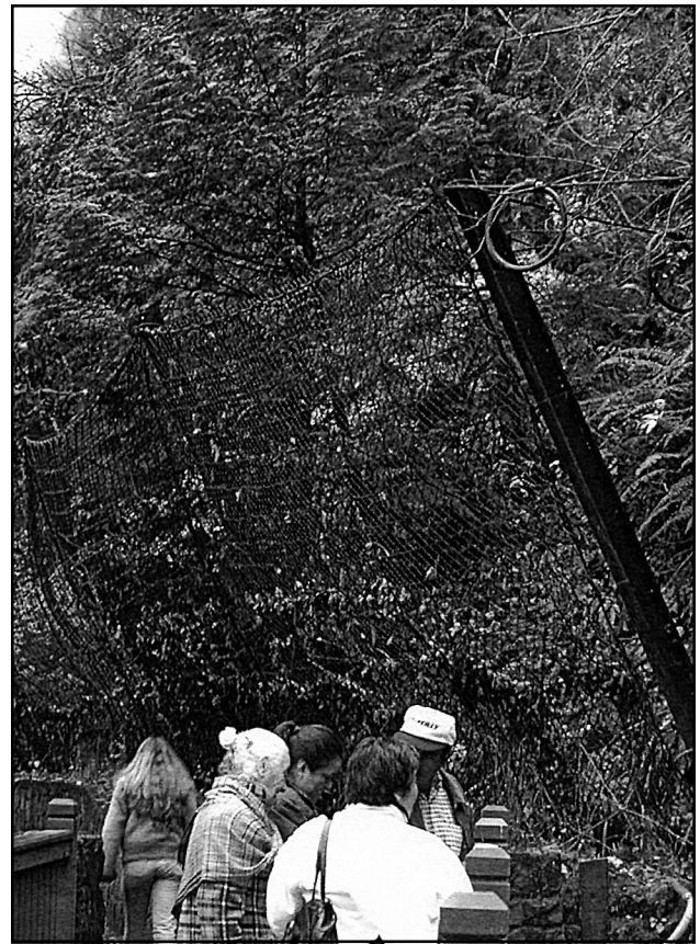
Figure 8. Multnomah Falls rock catchment net on the footpath to the bridge. This was installed by the U.S. Forest Service as a result of a tourist injury.
