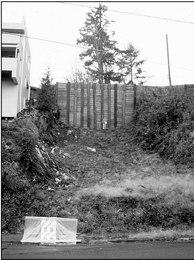
Figure 10. The soldier pile wall built at the top of the Canterbury Castle Landslide in the summer of 1996. It failed the following winter.
