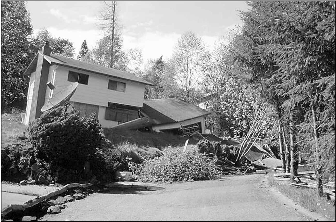
Figure 1: Destroyed house on the Aldercrest–Banyon Landslide in Kelso, Washington. Note the thrust of soil under the house.
