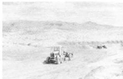
Figure 7. Material from the flat-lying bed being loosened and windrowed by a disk and scraper.
