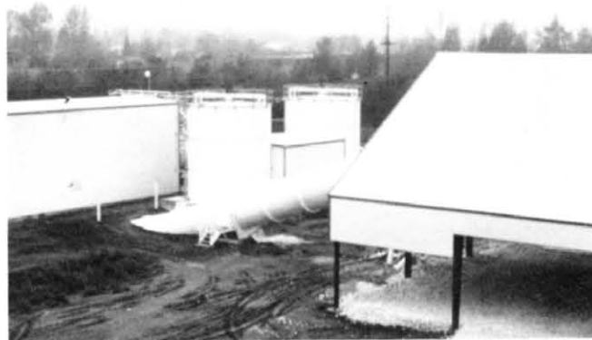
Figure 4. Columbia River Carbonates produces fine- and ultra-fine-ground calcium carbonate at this plant in Cowlitz County. The enclosed conveyor system at the plant reduces contamination of the white rock. Photo courtesy of Columbia River Carbonates.
