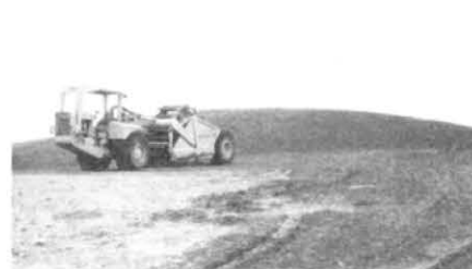
Figure 8. Three- or 4-in. lifts of air-dried bentonite being removed and loaded into trucks with a wheeled elevator and moved to stockpiles.
