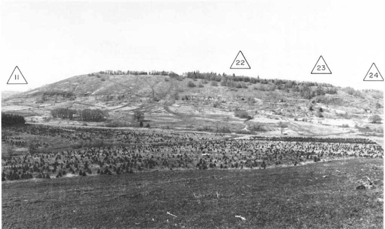
Figure 4a. Coffin Butte. Quarry sites 11, 22, 23, and 24 have been developed in Siletz River Volcanics. Although not apparent from this angle, sites 22 and 23 are filled with water. Note motorcycle trails crisscrossing ridge.
