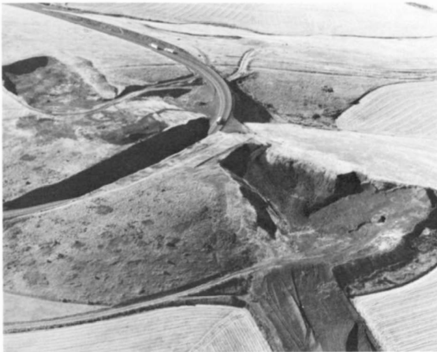
Photo 2. Columbia River Basalt from quarries and roadcut was used for construction of Highway I-80 at Cabbage Hill east of Pendleton.
