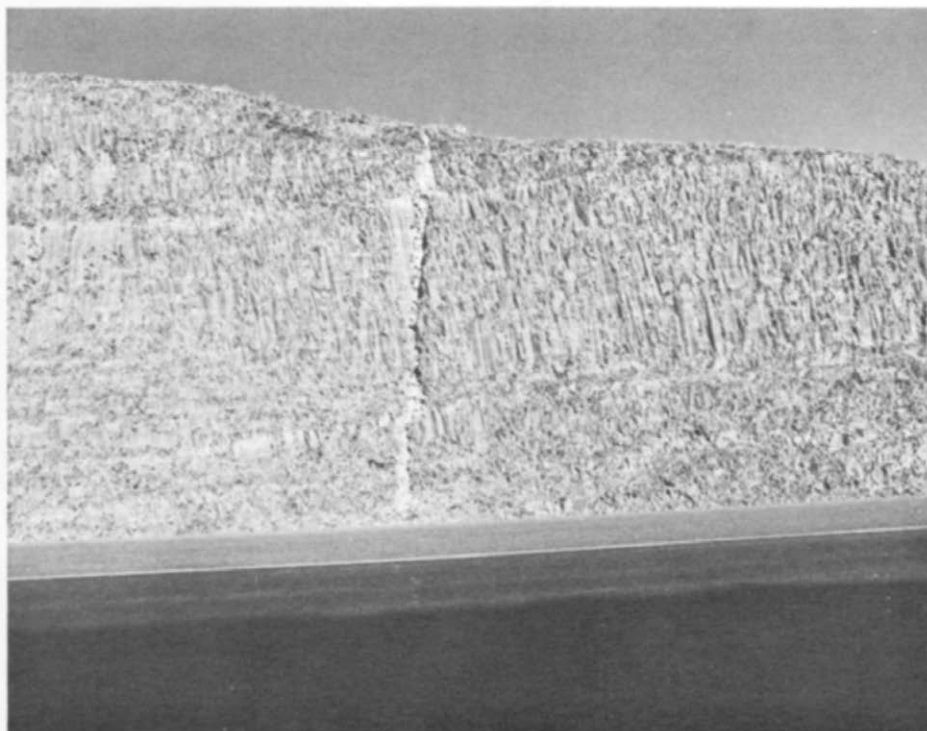
Photo 8. Columbia River Basalt exposed in roadcut on Highway I-80 at Cabbage Hill. Note the fine columnar joint pattern. This rock makes excellent crushed aggregate for base course and surfacing.
