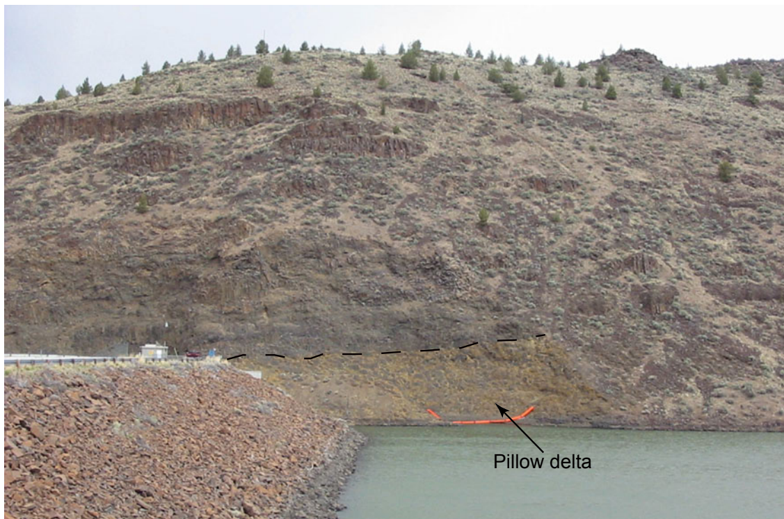
Figure 5. Pillow delta exposed at the base of a thick section of Prineville Basalt along the right abutment of Bowman Dam near stop 3.
