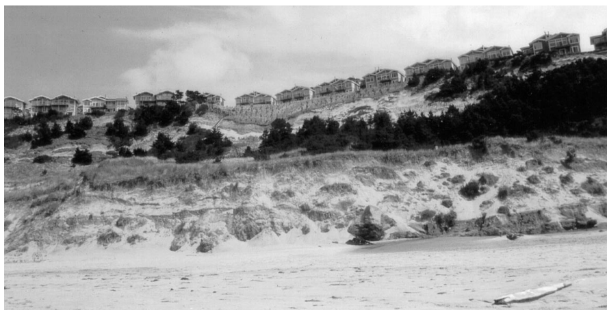
Erosion of dune sand at The Capes development led to landsliding which endangered homes.
