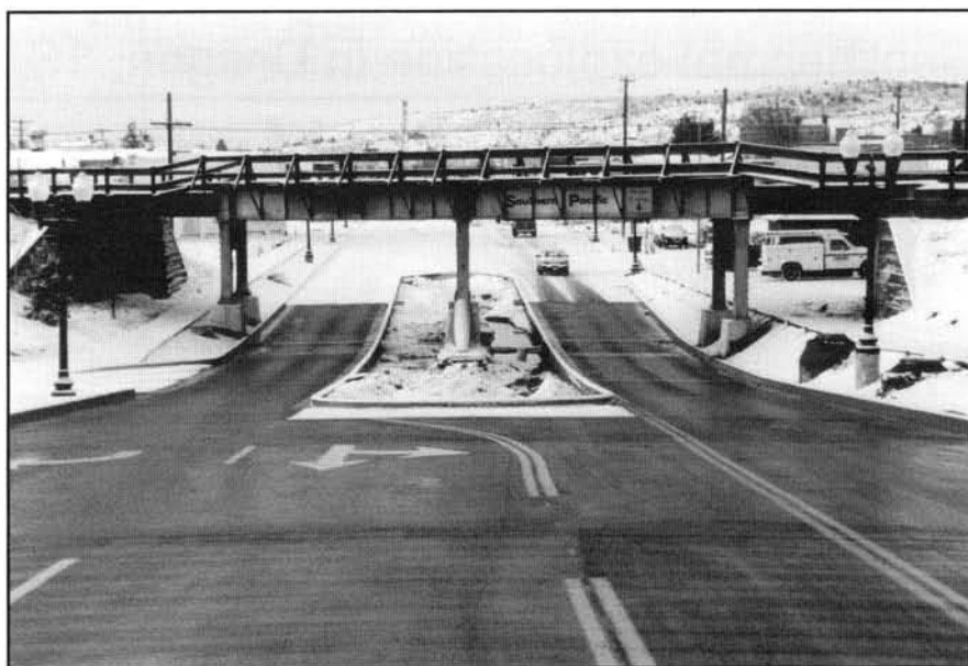
Oregon Department of Transportation project on Esplanade in Klamath Falls. Buried warm-water pipes keep snow melted. Photo courtesy John Lund, Geo-Heat Center, Oregon Institute of Technology.
