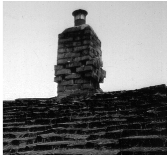
Chimneys, usually built of unreinforced masonry, show the most common type of damage caused by the 1993 Scotts Mills earthquake. Photos show house near Molalla on left and roof of authors' home near Scotts Mills (right). Photos courtesy of Doug Eaton.
