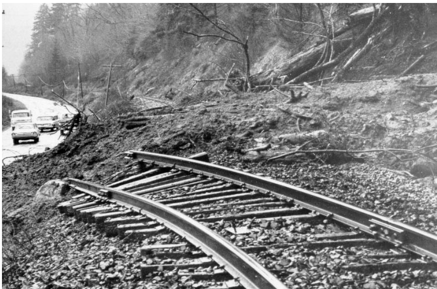
Bent railroad tracks and blocked coastal road at Mapleton, Oregon, reflect the power of a mudflow there in 1964.
