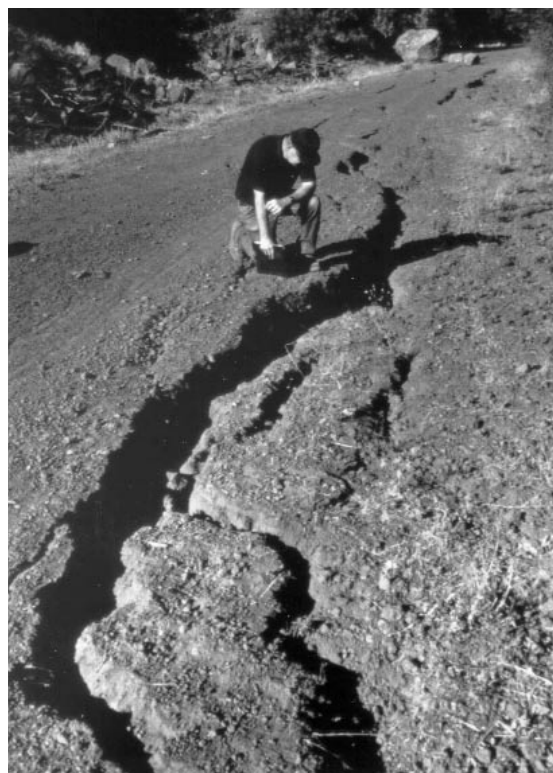
The huge boulder above was dislodged and fell on Highway 140 west of Howard Bay at Upper Klamath Lake during the 1993 Klamath Falls earthquake, which also produced a rotational slump and its associated crescent-shaped cracks in the roadbed nearby (right).
