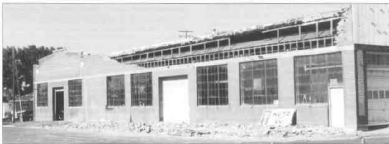
Typical damage to a parapet made of unreinforced masonry (URM), caused by the Klamath Falls earthquakes of 1993.
