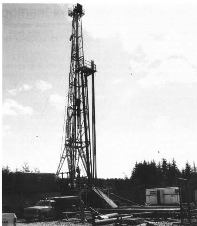
At the Northwest Natural Gas well IW 23d-3, an injection-withdrawal well at the Flora gas storage pool, preparations are in progress to install surface casing. The surface casing consists of large-diameter pipe that is cemented in the well for protecting fresh-water resources, anchoring blowout-prevention equipment, and maintaining the integrity of the surface hole.
