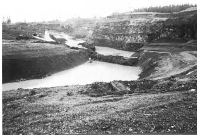
Morse Brothers, Inc., Progress Quarry operation near Beaverton, Washington County. Mined-out quarry area is being back-filled with about 600,000 yds of clean material for protection of ground water.
