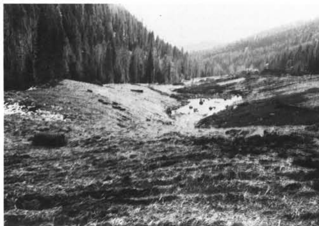
The same Bonnanza Mining operation area as in photo above, after completion of backfilling. View is to the south. Ponded area in background is a newly created artificial wetland area.
