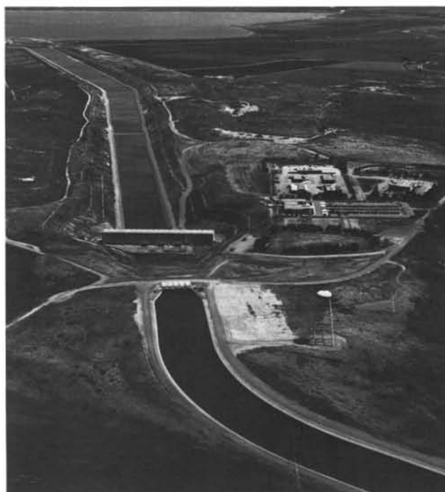
Harvey O. Banks delta pumping plant, southern area of the Sacramento-San Joaquin delta, California, is shown in the distance. This plant marks the beginning of the California Aqueduct, the largest aqueduct system in the world. Over 8 million \text{yd}^3 of unreinforced concrete was used, and much of the aqueduct is 64 ft wide at the top, 32 ft deep, and 40 ft wide at the base. The average thickness of concrete is about 4 in. Photo courtesy of the California Department of Water Resources.
