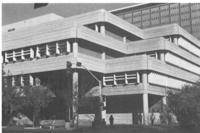
Concrete state office building in Sacramento, California. The concrete walls are nearly 7 in. thick. The high mass enables the concrete to store and release large amounts of thermal energy. In other words, concrete is used to moderate temperature swings and save on heating and cooling costs. In the hot Sacramento summers, the interior walls absorb and store heat during the day and radiate it at night. The thick concrete walls and floors help maintain a steady interior temperature year-round.
