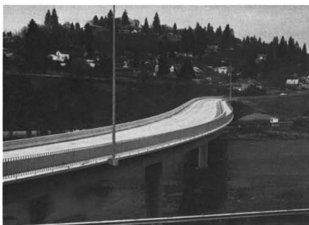
Hood River Bridge, Hood River, Oregon. Reversing 10° curves were used in this project to connect roads running on opposite sides of Hood River. Approximately 3,000 yd 3 of concrete were used, cast in place and post-tensioned. Photo courtesy of the Oregon Concrete and Aggregate Producers Association (OCAPA).
