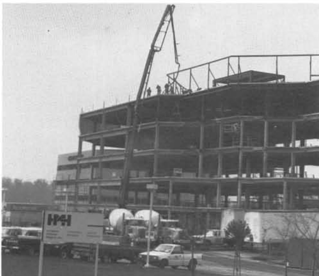
Concrete floor panel being placed by means of a tremie line. The concrete was made in a nearby batch plant, transported to the construction site by ready-mix trucks (seen at the base of the building), pneumatically pumped five stories high, and then placed into position by workers.
