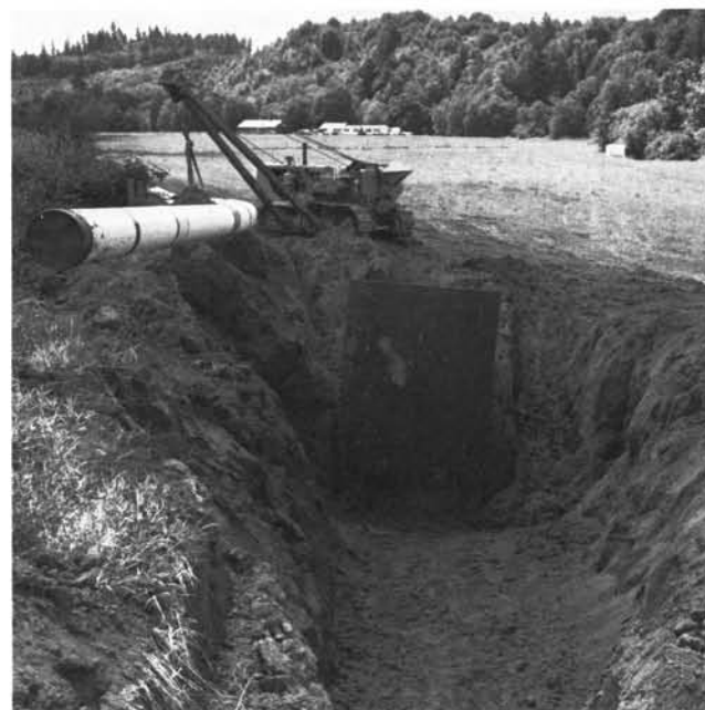
Construction of Northwest Natural Gas Company feeder pipeline just east of Mist.
