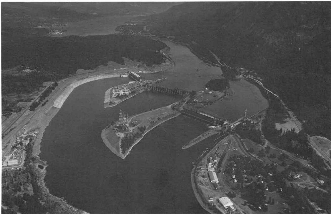
Bonneville Lock and Dam on the Columbia River, approximately 30 mi east of Portland, Oregon, connecting the Oregon and Washington sides of the river over a distance of about three-quarters of a mile. Built originally between 1933 and 1937 and enlarged in the early 1970's, the dam now combines the oldest and newest federal power plants on the Columbia. Lake Bonneville, the 48-mi-long reservoir impounded by the dam, is the first in a series of navigable lakes that are part of a water highway running 470 mi from the Pacific Ocean to Lewiston, Idaho. The Bonneville Lock and Dam project was placed on the National Register of Historic Places in 1986 and has been designated as a National Historic Landmark. Enormous quantities of concrete were used in this mass-concrete construction. Photo courtesy of U.S. Army Corps of Engineers, Portland District.
