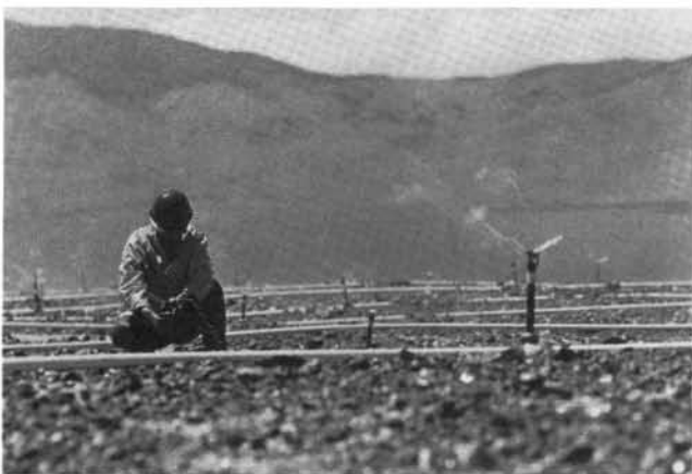
Cyanide solution being applied on heap leach pad at Atlas Mine. Photo courtesy of Atlas Gold Mining, Inc.
