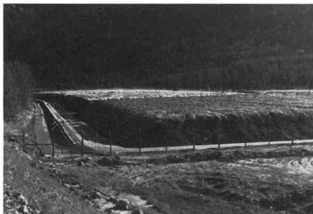
Heap leach pad in production. Only the section in background is currently being sprinkled with cyanide solution.
