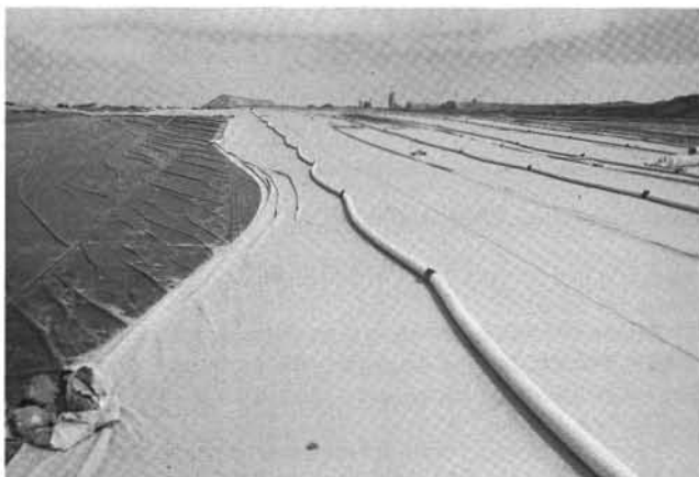
Base preparation of heap leach pad. On a slightly inclined surface, an impermeable plastic sheet (darker in color) is covered with a highly permeable synthetic material (lighter color). The permeable sheet and the perforated pipes serve to drain off the leaching solution after it has moved from the top to the bottom of the ore pile and become "pregnant." Under the impermeable sheet and not visible in the picture, a leak detection system is installed.
