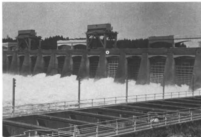
Spillway of Bonneville Dam (photo above). The term "mass concrete" used for this kind of construction refers to the fact that the concrete in these structures often is several feet thick. Photo courtesy of Bonneville Power Administration.
