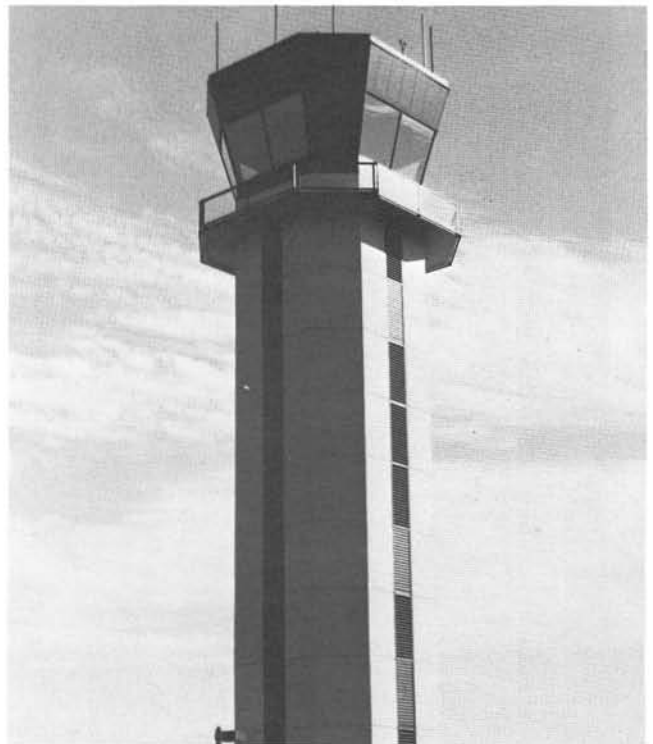
Airport control tower at Mahlon-Sweet Airport in Eugene, Oregon. Precast concrete is used in this construction, and the design can easily be repeated at other locations. Photo courtesy OCAPA.
