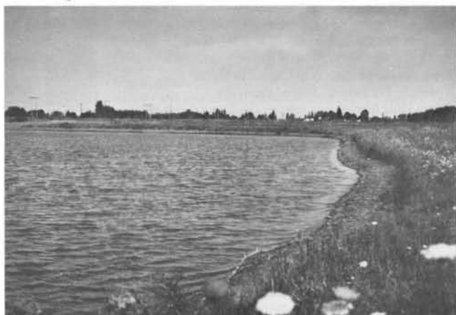
Oregon State Highway Division reclamation site near Junction City. The 10-acre lake, open to public fishing, has a "drown-proofed" shoreline, i.e., a shallow 3:1 slope extending 18 ft out from water's edge into lake. This also encourages growth of aquatic plants.
