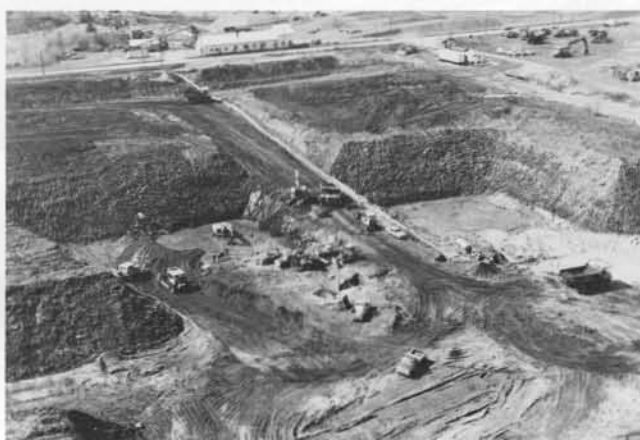
Excavation through landfill to base of former mined area for foundation of county headquarters building. (State Highway Division air photo)
