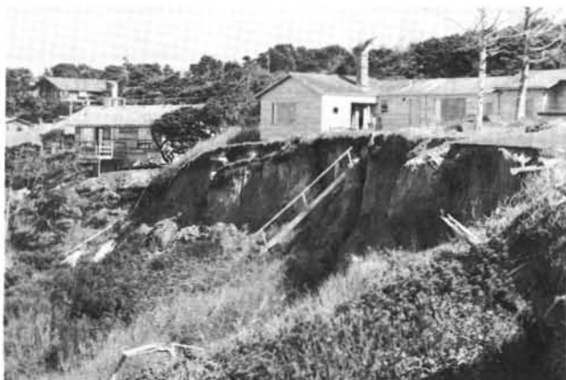
Active compound rotational slump (Reach 5, Map 12, Landslide 3 on strip map) on west side of Park Drive, in the vicinity of N. 14th St., Newport.
