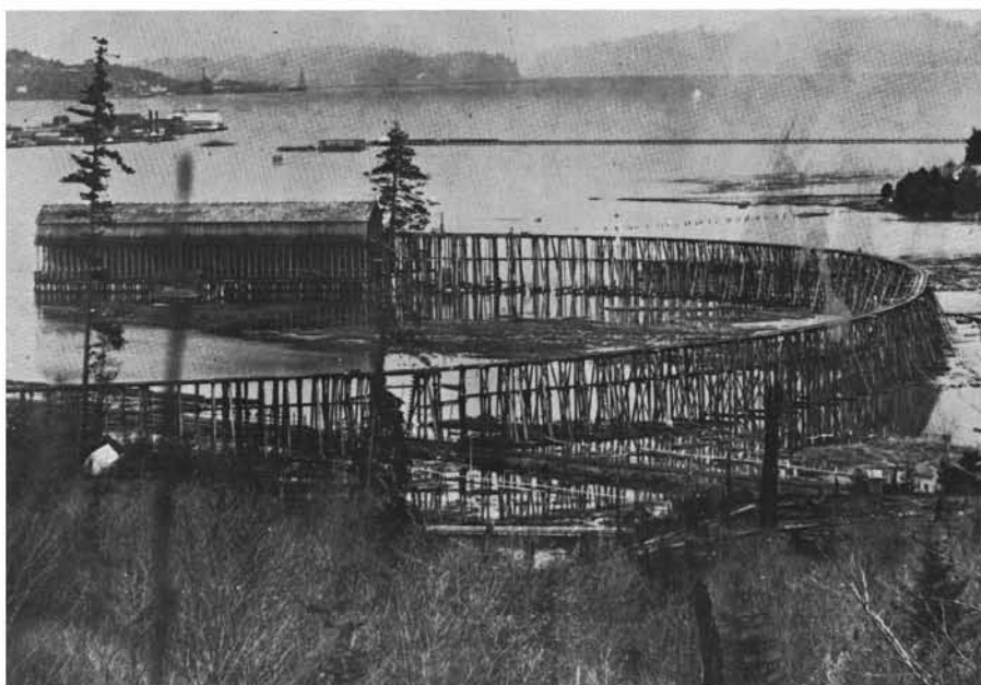
Figure 5c. Libby coal bunker on Coalbank Slough. From facilities such as these, coal was loaded onto ships and transported to the San Francisco Bay area. (Photo courtesy Jack's Photo Service, Coos Bay)
