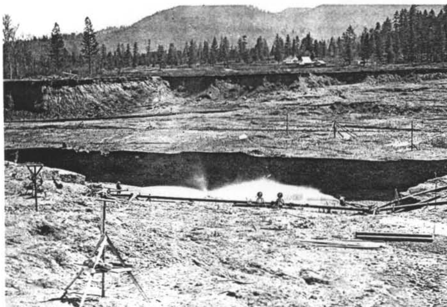
Figure 7. Giants similar to those described at checkpoint 28. These giants were operated in Josephine County, but similar ones were used in placer operations in the Bohemia district.
