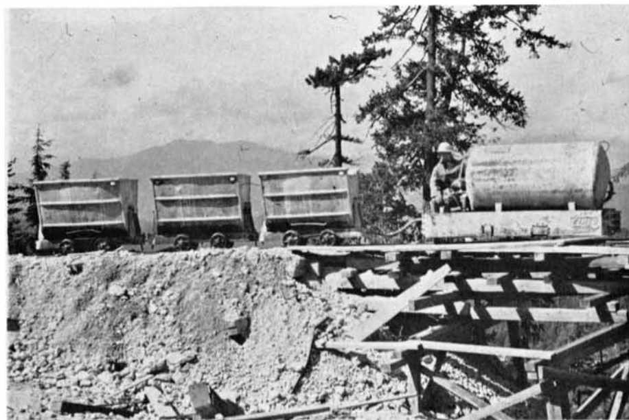
Figure 13. Three-car, compressed-air driven tram that ran from 1,000 level of Musick mine during diamond-drilling exploration program that included the Champion, Evening Star, Musick, and other mines in the Bohemia district.
