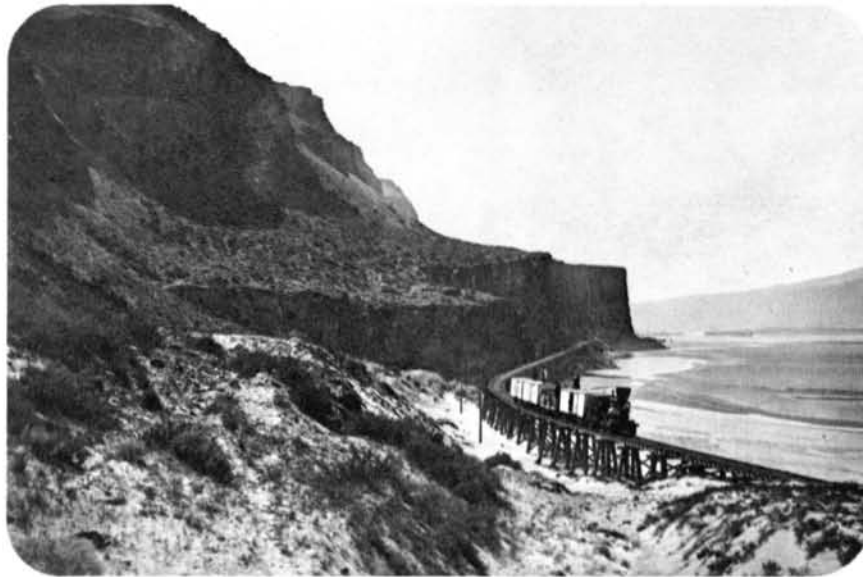
The difficulties of the portage above The Dalles and past Celilo Falls were lessened by the construction in 1863 of the 15-mile narrow-gauge "portage" railroad. Built on the Oregon side of the Columbia River at a reported cost of $50,000 per mile and in service until the 1880's, this railroad constituted an important link between the river boats plying the Columbia between Cascade Locks and The Dalles and those plying the up-river run from Celilo to Umatilla Landing and Lewiston. (Oregon Historical Society photograph)
