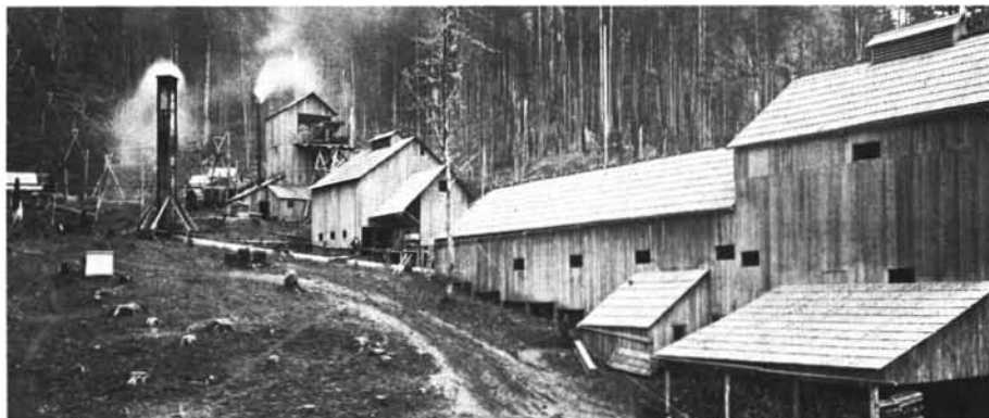
Figure 16. Black Butte mercury retort. Tramline in upper left transported ore downhill from mine to retort. Cinnabar containing mercury and sulfur was heated in rotary kiln to drive off sulfur. Free mercury left behind was condensed as quicksilver. Photo courtesy Daniel Mills.
