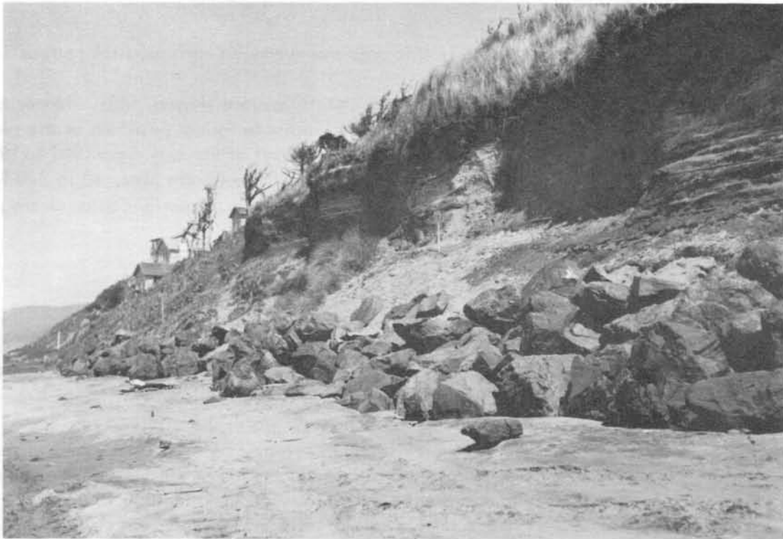
Figure 15. Low-cost preventive measures: riprap and "keep off" signs at Oceanlake (Lincoln City).
