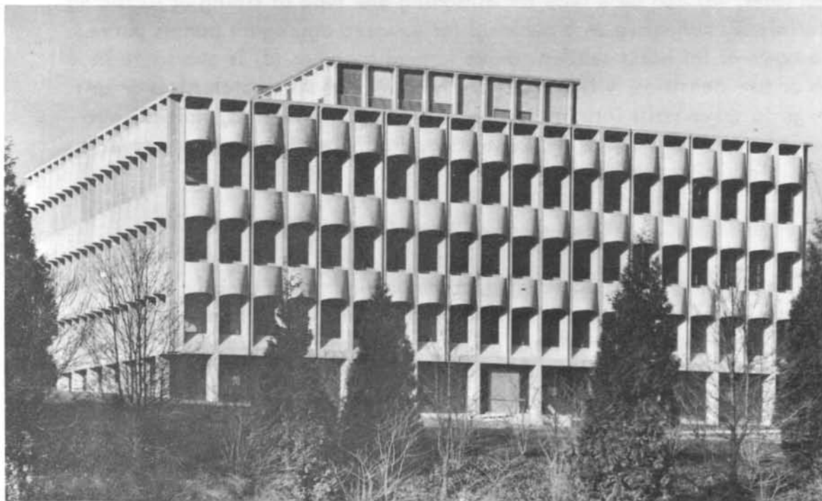
IBM Bldg., 2000 S. W. 1st Ave. (top). Thirty-eight smooth-surfaced concrete panels 12 feet wide and four floors high cover the structure and support the outer perimeter of the floors. Panels were cast in Tacoma and trucked to site. (Photo by W. H. Grand)
