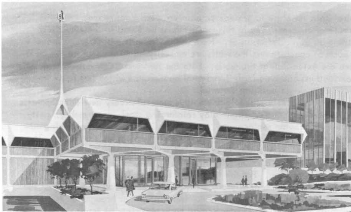
Pioneer Broadcasting Bldg. (KGW-TV). Splayed poured-in-place concrete posts support the second floor, which features thin-shell concrete sunscreens. Uncompleted building is at 1500 S. W. Jefferson St. (Photo by Alan Hicks)
