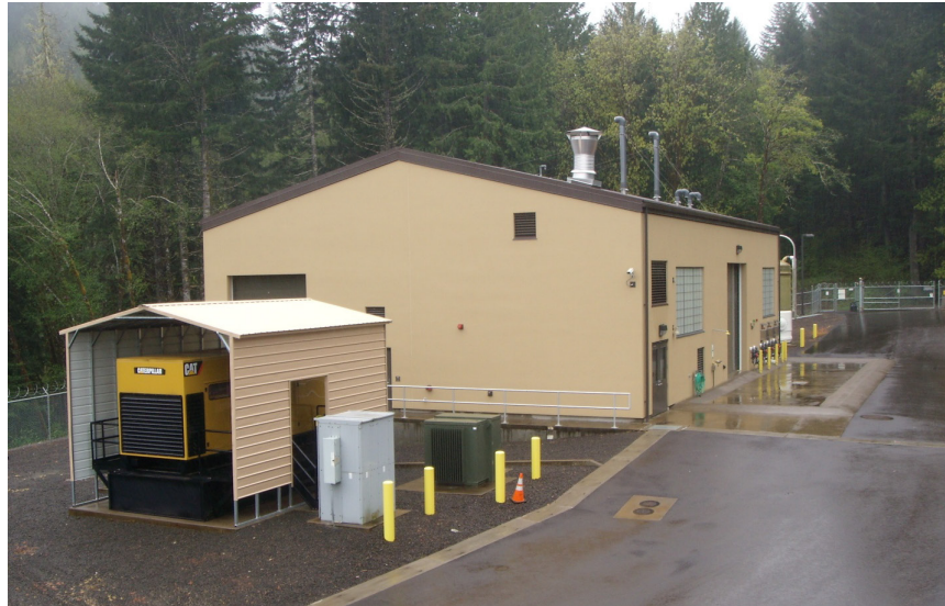
Figure 2-24. McMinnville Water and Light water treatment plant showing the chemical building and emergency generator (foreground). (Photo by Yumei Wang)
