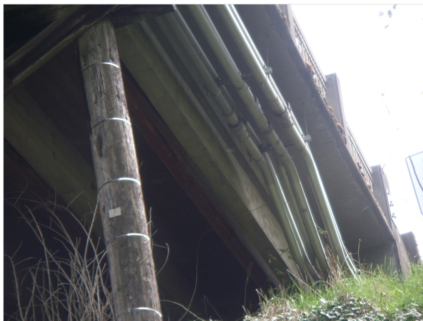
Figure 2-32. Close-up of the south abutment of Three Mile Lane bridge showing colocated lifelines, including a major telecommunication line. Earthquake-induced bridge damage could disrupt communication services. (Photo by Yumei Wang)
