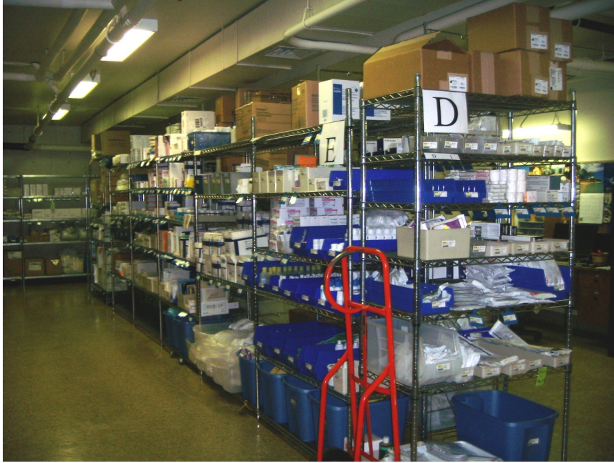
Figure 2-17. Lincoln City (Samaritan North Lincoln) hospital with contents damage potential, such as medical supplies falling from shelves that have not been seismically secured. (Photo by Yumei Wang)
