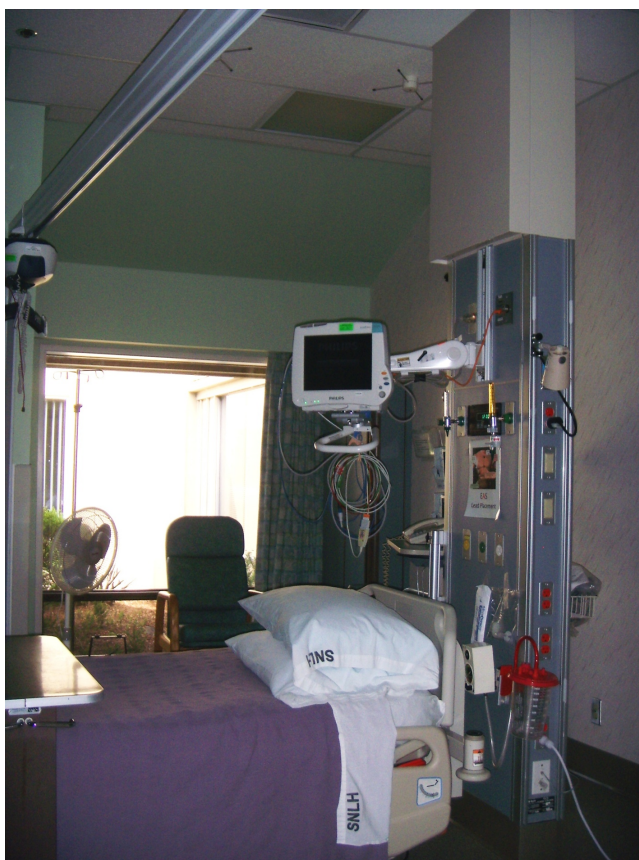
Figure 2-16. Lincoln City (Samaritan North Lincoln) hospital patient room with nonstructural damage potential, such as falling suspended ceiling tiles and medical equipment. (Photo by Yumei Wang)
