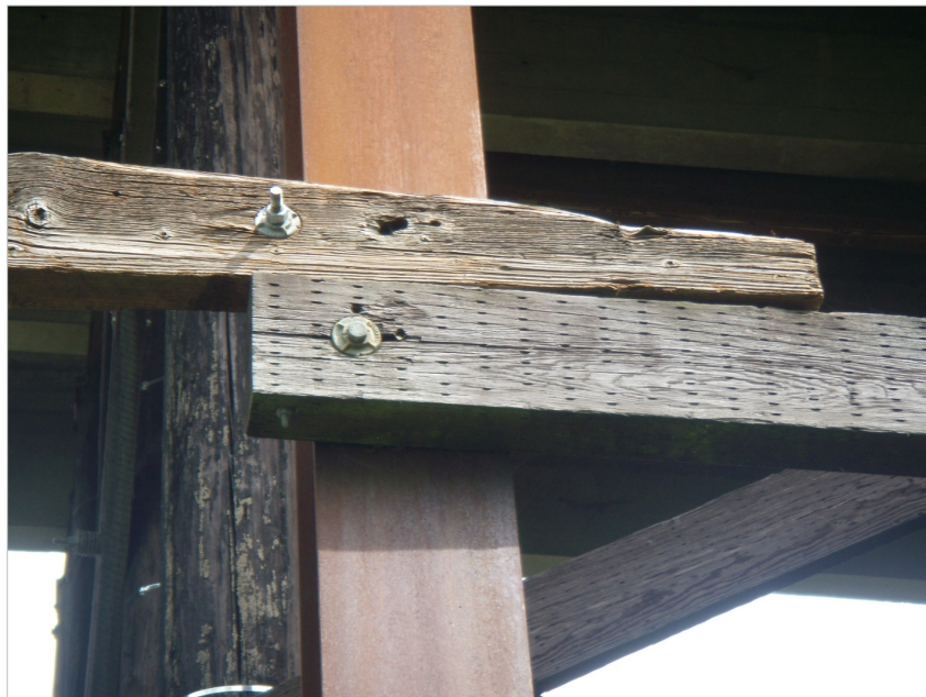
Figure 2-31. Close-up of Three Mile Lane bridge showing various ages and types of materials in the substructure, including steel and wood. This photo shows the inadequate seismic design, construction, and maintenance, including split timber members. As supported by our analyses, it will likely be inoperable after a major earthquake. (Photo by Yumei Wang)
