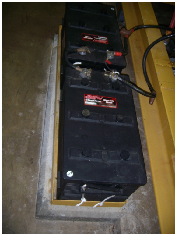
Figure 2-22. Batteries for the emergency generator at the City of Lincoln City water treatment plant. The batteries have not been seismically restrained and may not operate the generator after a Cascadia earthquake. (Photo by Yumei Wang)
