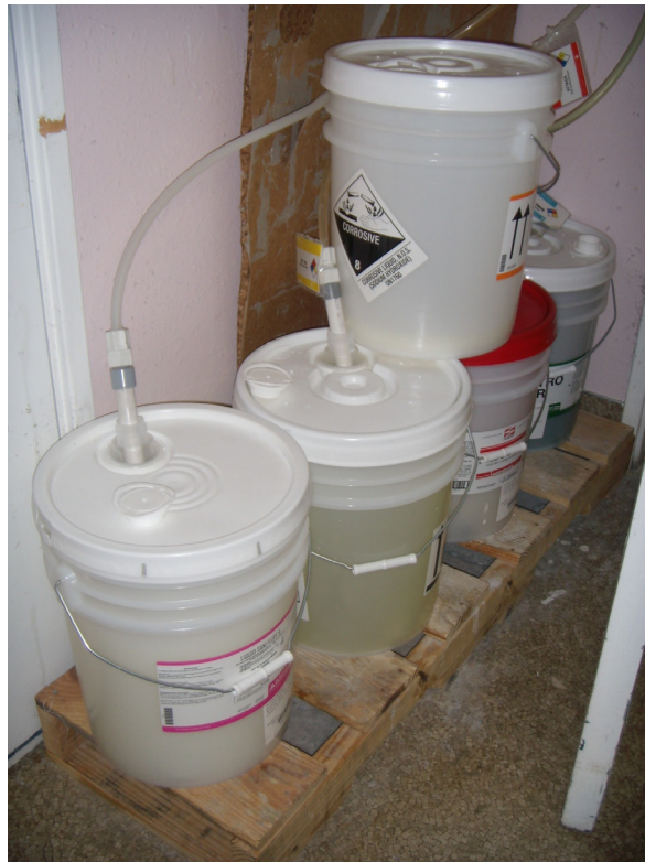
Figure 2-18. Lincoln City (Samaritan North Lincoln) hospital has potentially hazardous chemicals that are not secured to withstand earthquake shaking and may spill. (Photo by Yumei Wang)
