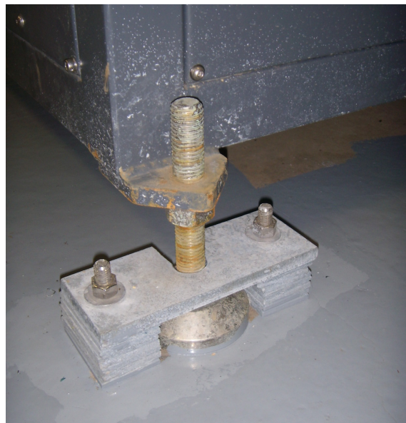
Figure 2-25. McMinnville Water and Light water treatment plant showing equipment without adequate seismic anchorage. Note the missing upper nut on center bolt. Proper seismic restraints of mechanical equipment may require seismic analyses. (Photo by Yumei Wang)
