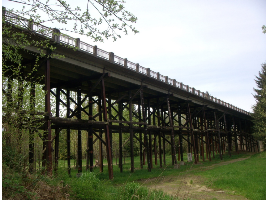
Figure 2-30. The 1951 Three Mile Lane bridge crosses the Yamhill River and connects downtown McMinnville and the hospital. It is in poor condition and has a telecommunication main line colocated on it. (Photo by Yumei Wang)
