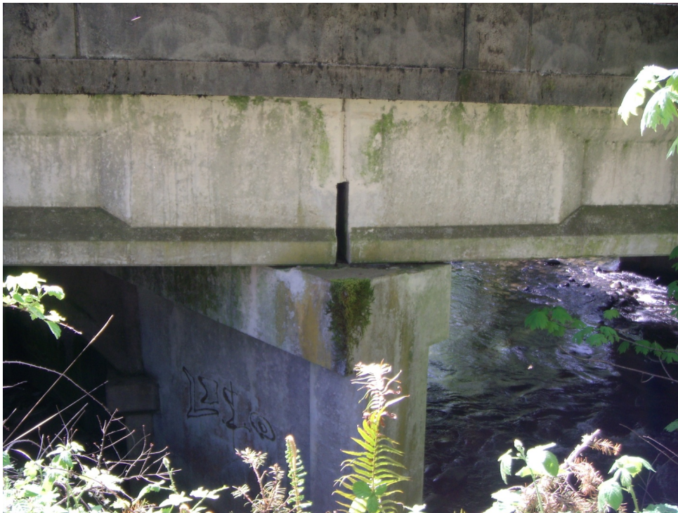
Figure 2-29. Bear Creek bridge on Highway 18 is expected to incur major damage during a Cascadia earthquake (Nako and others, 2009). One seismic deficiency relates to the inadequate width of the bearing seats; the bridge deck girders could slip off their supports during horizontal ground motions and render the bridge inoperable. (Photo by Yumei Wang)
