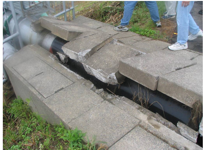
Figure 2-6. Water transmission pipeline failure at a river crossing in the 2007 Kashiwazaki, Japan earthquake. (Photo by Yumei Wang)
