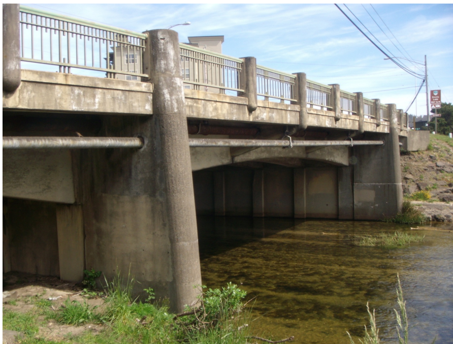
Figure 2-33. A 10-inch-diameter water transmission pipeline is colocated on the D River bridge on coastal Highway 101. This bridge is expected to experience tsunami inundation; in that event the pipeline is expected to incur breaks caused by bridge damage. A new, more reliable transmission pipe will be constructed under the river. (Photo by Yumei Wang)
