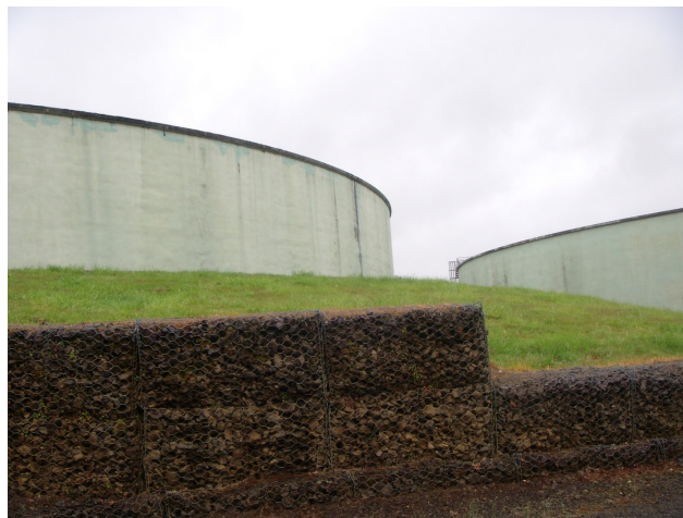
Figure 2-27. McMinnville Water and Light showing two of the four Fox Ridge reservoirs. These are the pre-stressed concrete tanks. (Photo by Yumei Wang)
