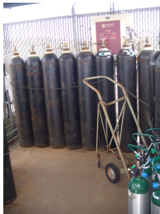
Figure 2-20. Medical gasses at McMinnville hospital (Willamette Valley Medical Center) are stored without seismic considerations. (Photo by Yumei Wang)
