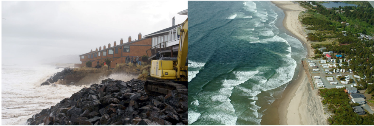
Figure 3-8. (left) Storm waves damage a riprap structure during a moderate storm in January 2008 in the community of Neskowin (Photo: A. Thibault, 2008); (Right) A rip embayment sets up immediately in front of the Shorewood RV park, Twin Rocks, enabling waves to attack the structure during storms. (Photo: D. Best, 2007)
