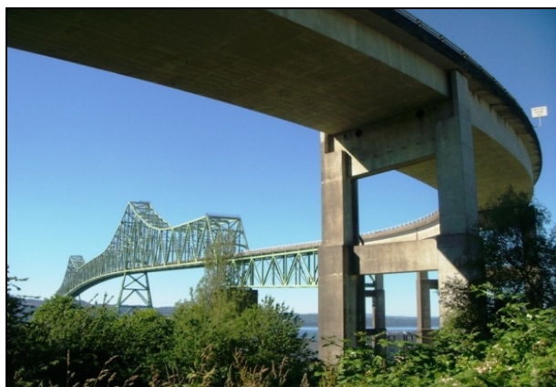
The approach (foreground) to the 1966 Astoria-Megler Bridge that spans the Columbia River has major structural deficiencies that could lead to a collapse following an earthquake. Damaged bridge sections could block waterway access to the CEI Hub. (DOGAMI photo)
