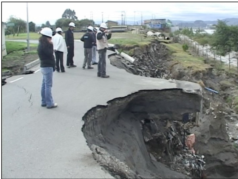
Figure 59: An example of damaged water transmission pipelines in the 2010 Chile earthquake. This limited water availability for emergency response as well as for businesses and daily living. (Technical Council on Lifeline Earthquake Engineering - TCLEE, 2010)
