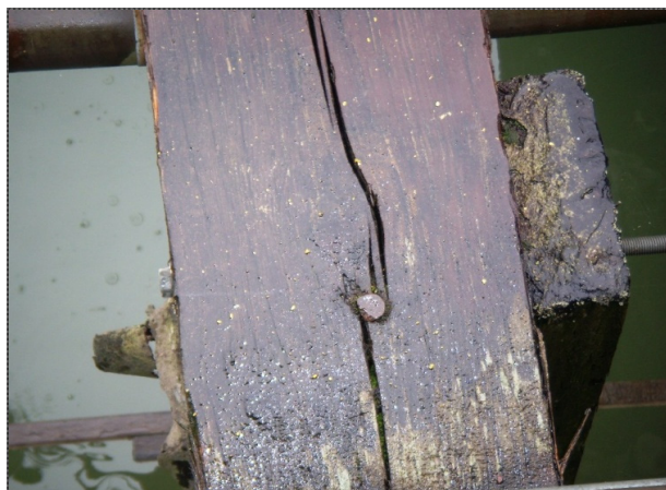
The connection on this pier in the CEI Hub appears to have deteriorated due to a split in the timber beam. This type of damage suggests that the condition of the structure may not be routinely monitored and maintained and that the overall pier is seismically vulnerable. (DOGAMI photo)
