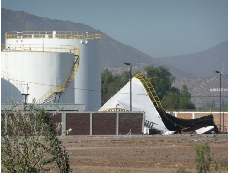
Figure 58: Structural damage to water tank located in fuel tank farm in Santiago from the 2010 Chile earthquake (Technical Council on Lifeline Earthquake Engineering - TCLEE)
