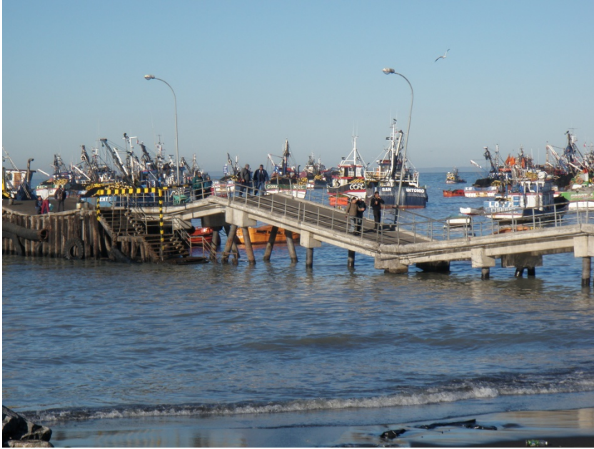
Figure 44: An example of a damaged pier in the 2010 Chile earthquake (Technical Council on Lifeline Earthquake Engineering – TCLEE - 2010)
