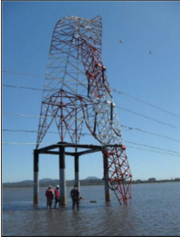
Figure 60: Structural damage to high voltage transmission tower located in river crossing in 2010 Chile earthquake. This limited electricity availability while temporary towers were installed (Technical Council on Lifeline Earthquake Engineering - TCLEE)
