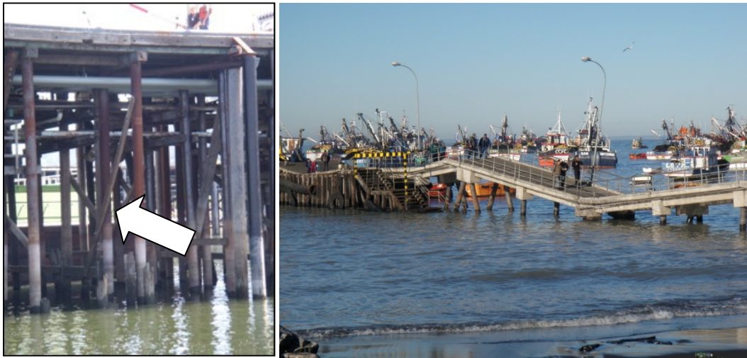
Left: Lateral timber bracing for steel plumb piles in the CEI Hub is considered inadequate by California's MOTEMS standards. (DOGAMI photo) Right: An example of a damaged pier in the 2010 Chile earthquake (Technical Council on Lifeline Earthquake Engineering – TCLEE, 2010)
