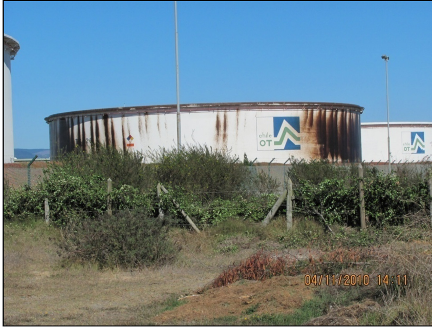
Figure 27: Sloshing of crude oil during the 2010 Chile earthquake. Note the black oil stains on the outside of the fuel tank. (Wang photo)
