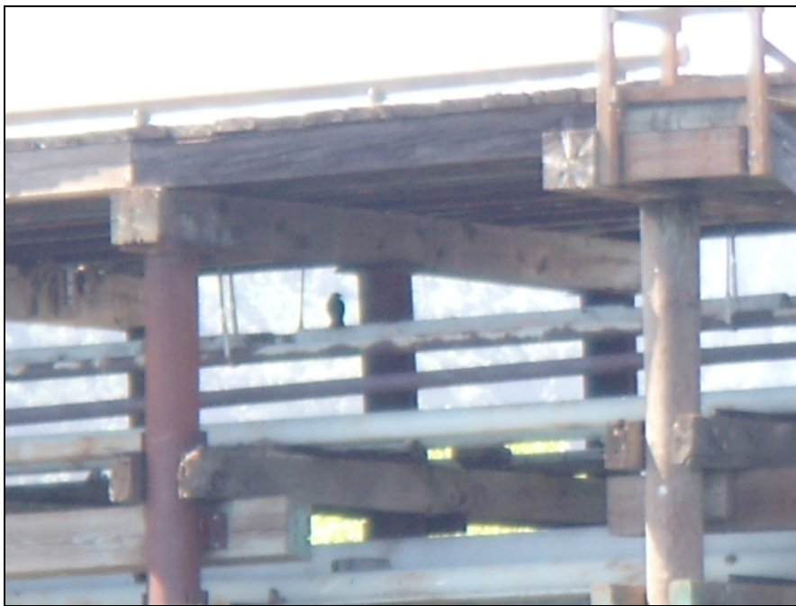
Figure 38: This photo shows generally poor condition of transverse beams supporting petroleum pipelines and cap beam in the CEI Hub. Notice the clockwise rotation of the pile cap beam in the center of the photo. (DOGAMI photo)
