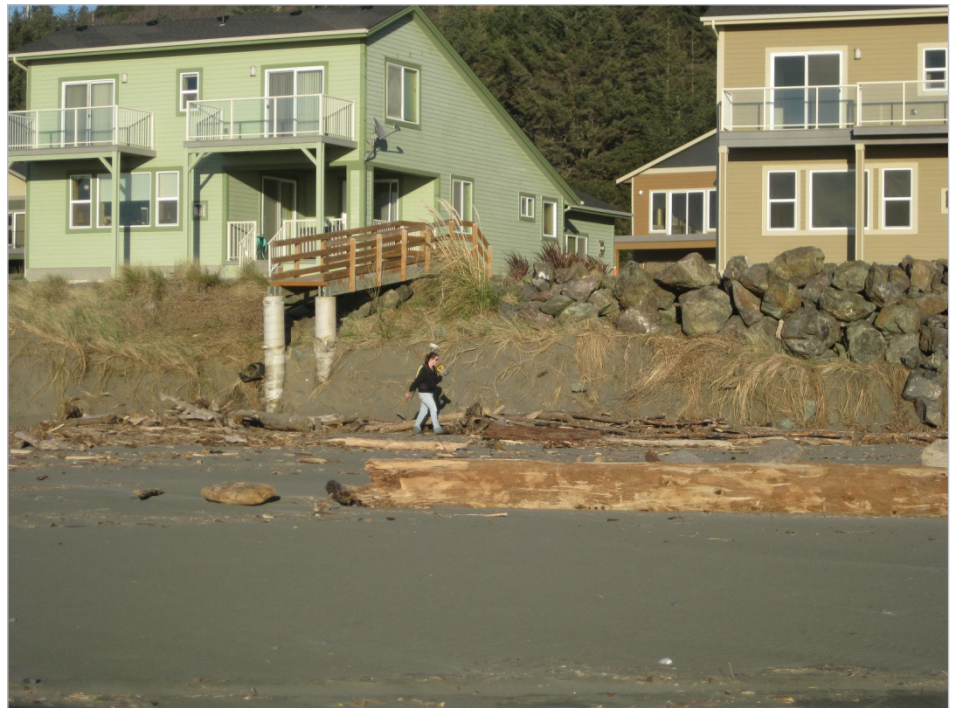
Figure 16. Homeowners placed riprap to mitigate erosion caused by a combination of Hunter Creek riverine channel erosion and wave runup and overtopping of the barrier beach. Photo shows DOGAMI geologist Laura Stimely surveying the toe of the erosion scarp.
