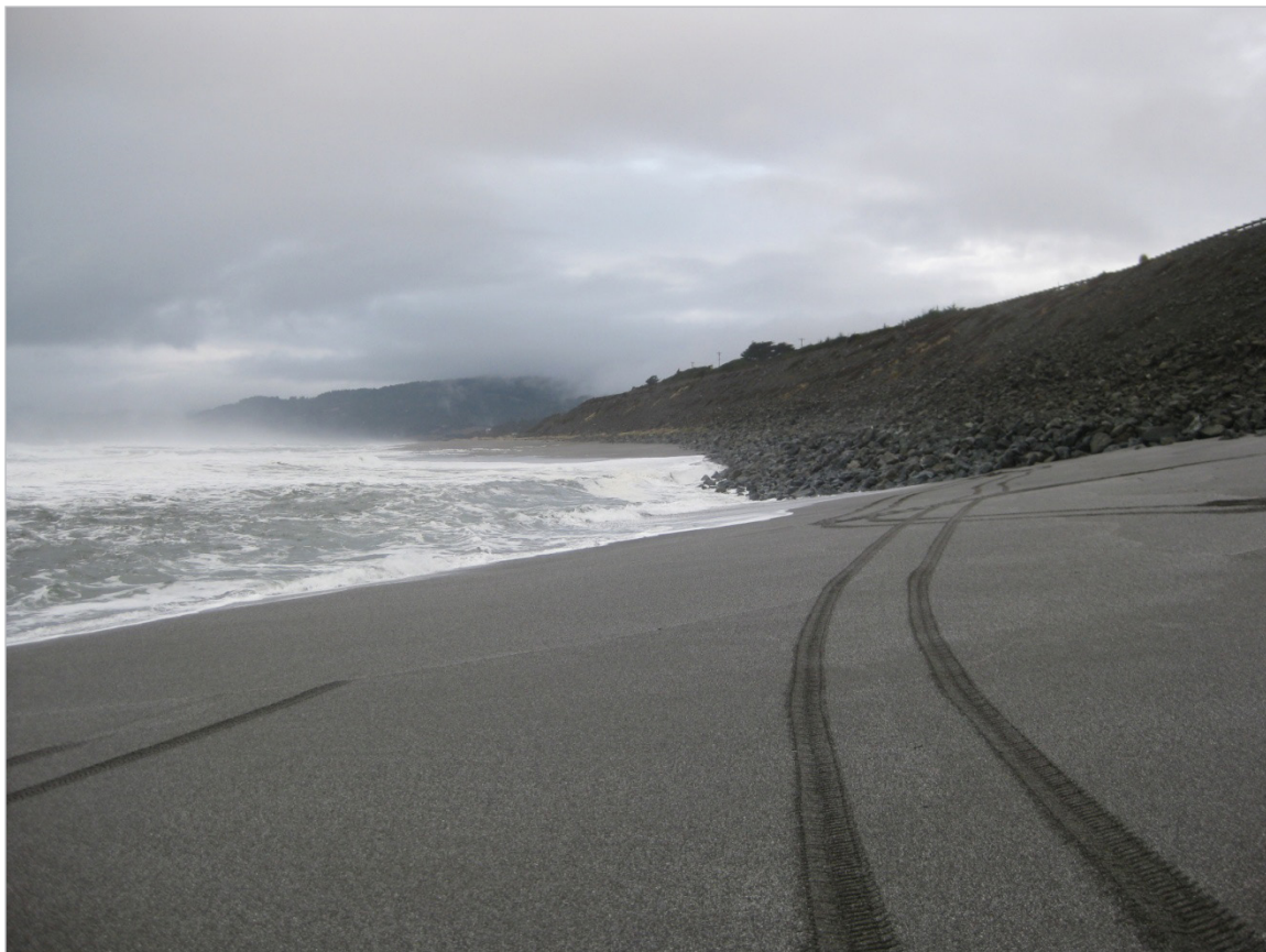
Figure 20. Development of a rip embayment adjacent to U.S. Highway 101 allows waves to directly attack the toe of the revetment. The photo was taken at low tide on February 16, 2011.
