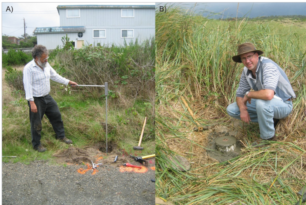
Figure 7. A) Installation of sectional aluminum rod topped by a 2.5-inch aluminum cap. B) The sectional rod and cap concreted in place.
