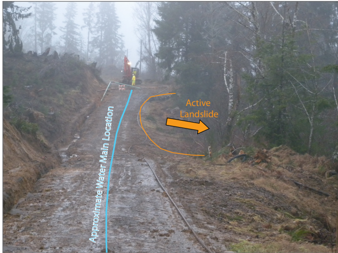
Figure 21. Photo showing the City of Astoria's potable water main proximity to an active landslide.
