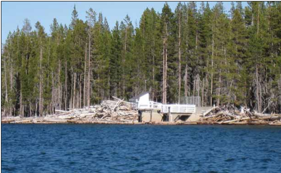
Figure 15B. Piles of driftwood in and around the Fourmile Lake Dam are depicted along with a fenced walkway that is joined to the dam and provides access to the submerged pipe that provides water to the Cascade Canal.
