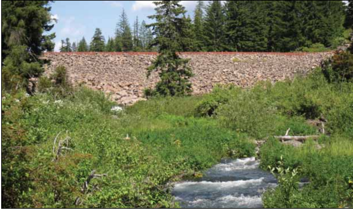
Figure 18A. The Fish Lake Dam, a predominantly boulder façade with a lining of very fine grained impermeable sediment on the reservoir side, was constructed near the headwaters of the North Fork of Little Butte Creek. Downstream of the dam the water flows west down the west flank of the Cascade Mountains to the White City – Medford area.
