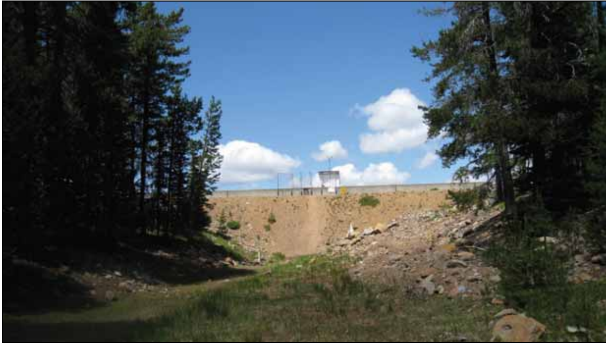
Figure 15A. This image is a view of the Fourmile Lake earthen dam. Water leaves Fourmile Lake in one of two ways (excluding infiltration and evaporation): either via the concrete overflow sluiceway, which is farther to the right in the image, or through a fixed diameter pipe that supplies all the water to the Cascade Canal and that is depicted below in Figure 15B.
