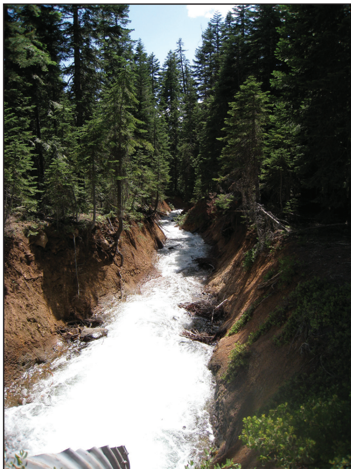
Figure 11D. A view of untypical water flow in the Cascade Canal after water exits a culvert under the access road that connects Oregon Route 140 to the Fourmile Lake USFS campground. This very turbulent flow in the canal causes severe erosion downstream from the culvert.
