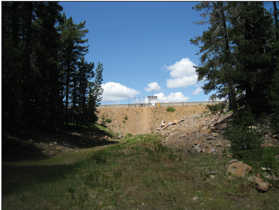
Figure 9. The earthen dam holds back Fourmile Lake. A concrete overflow structure farther to the right prevents water from over-topping the dam.
