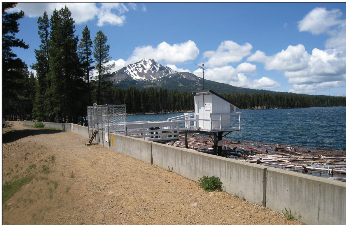
Figure 11A. This image was taken at the dam at Fourmile Lake and depicts the white wooden structure that sits atop the pipe that siphons off lake water and feeds it into the Cascade Canal. The drainpipe is located well below lake level in order to maintain a constant flow of water into the canal.
