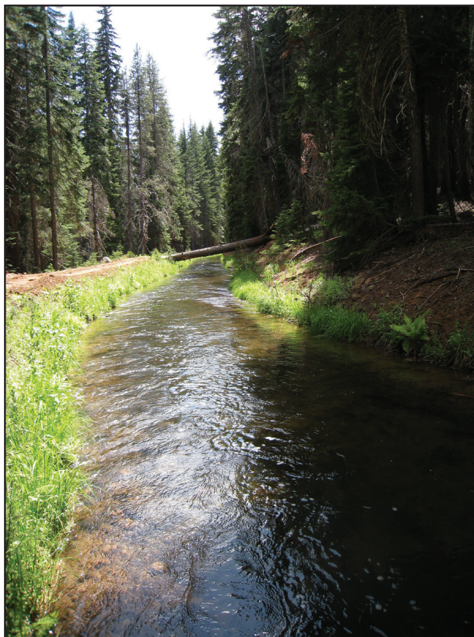
Figure 11B. This view of the Cascade Canal, taken a mile or so below Fourmile Lake dam, shows the typical canal. The canal is an unlined trench 3 to 4 m wide and 1 to 1.5 m deep.
