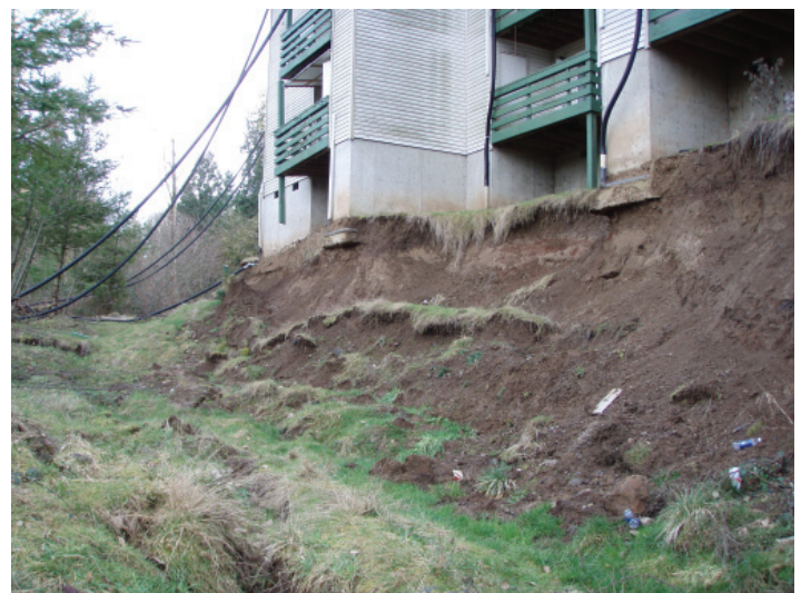
Figure 8. Photographs showing scarps along the crest of the toe of the large Newell Creek Apartment landslide from (left) 2006 and (right) 2007.
