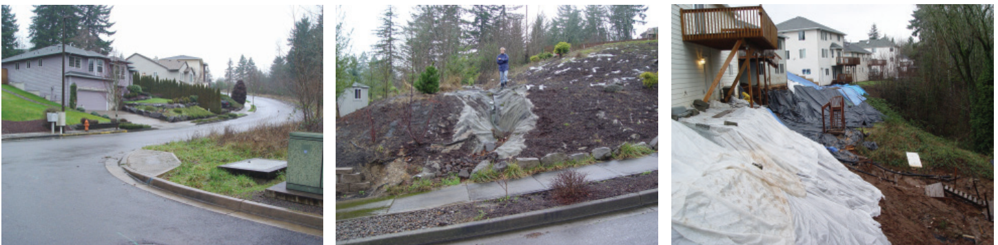
Figure 13. Barclay Hills subdivision. (left) In 1996 the toe of the slide moved 25 cm (10 in) and disconnected the sewage pumping station. (center) Upper part of the slide shows movement at the scarp. (right) In December 2006 the backyards of three homes at the end of Barclay Hills Drive slid away.
