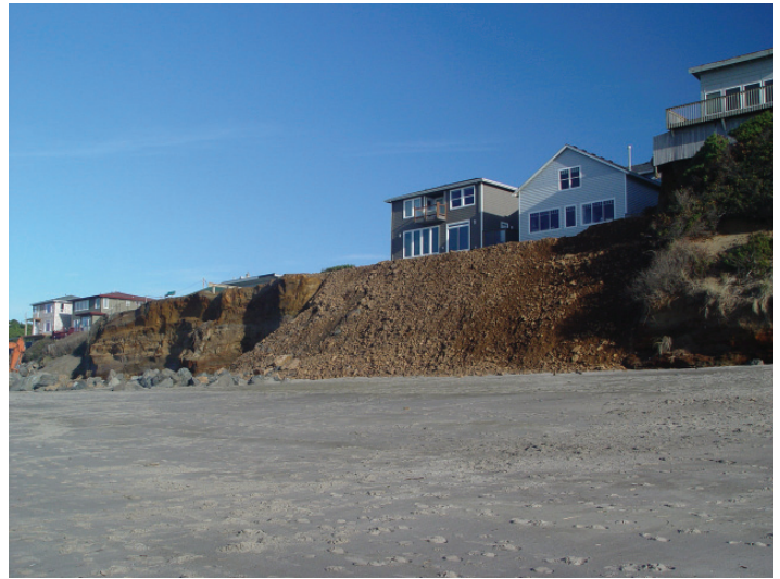
Figure 26. Site photograph in 2007 of rockfill and rip-rap along the beach (western) side.
