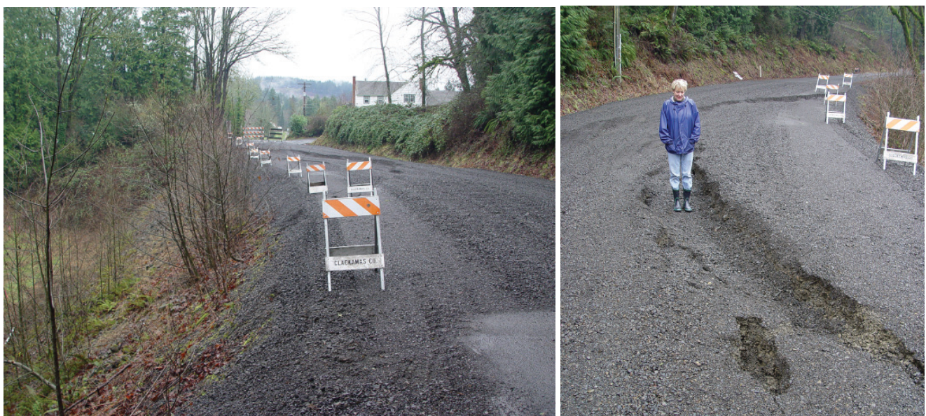
Figure 22. Site photographs in 2007 show fill failure just one month after the road was repaired for the third time.
