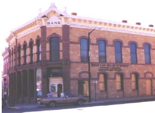
Example of a Bearing Wall Structure
