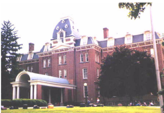
Figure E-50 East coast URM bearing-wall building.
