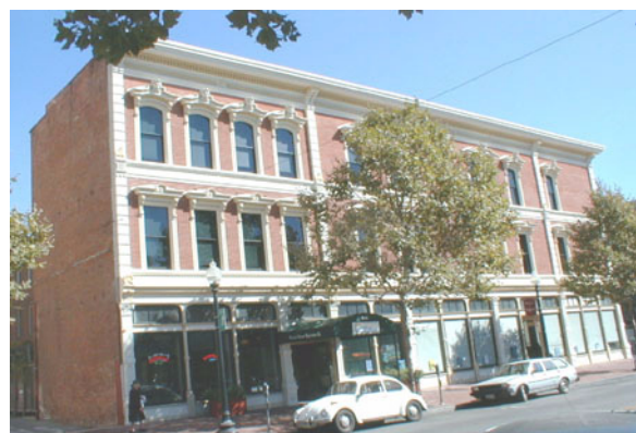
Figure E-51 West coast URM bearing-wall building.
