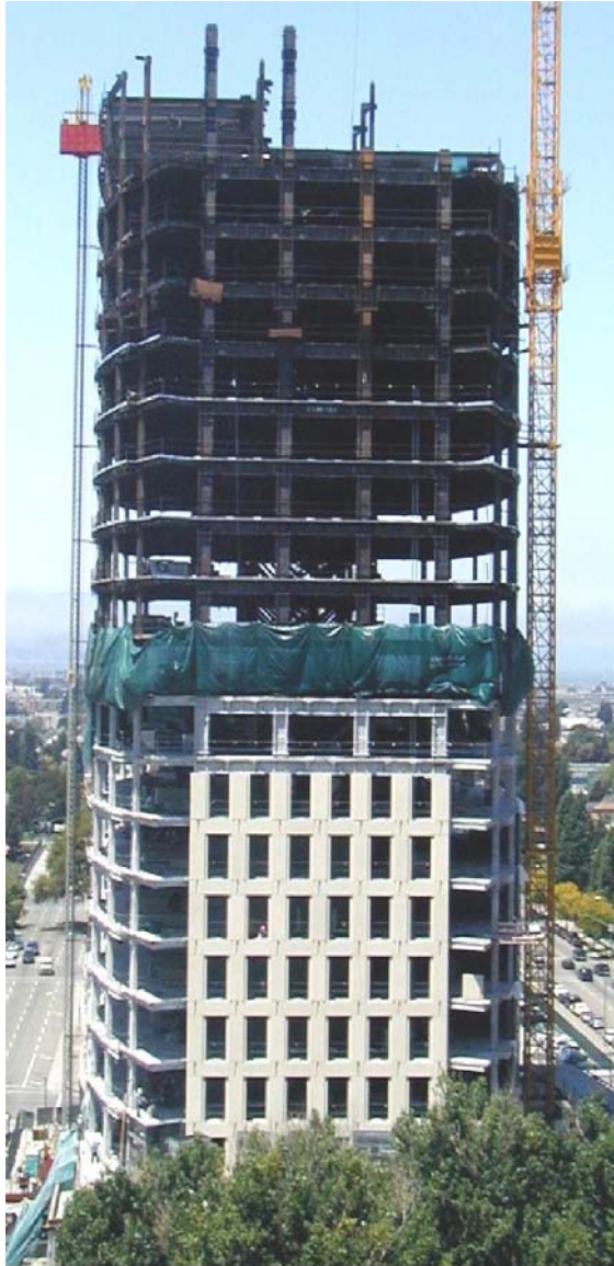
a. Building above is a high-rise steel dual system – moment frame (heavy columns and beams on upper facade) with bracing around elevator core. Fireproofing is being applied to steel at mid-height (inside the shroud) and precast facade elements are being attached to frame in lower stories.
