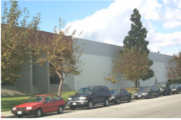
Figure E-36 Tilt-up industrial building, 1970s.
