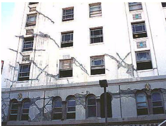
Figure E-32 Shear-wall damage, 1989 Loma Prieta earthquake.
