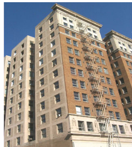
Figure E-33 Concrete frame with URM infill.
