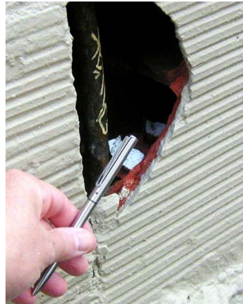
Figure D-14 Hollow clay tile wall with punctured tile.
