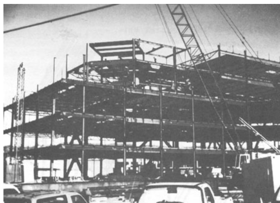
Figure E-13 Braced steel frame, with chevron and diagonal braces. The braces and steel frames are usually covered by finish material after the steel is erected.
