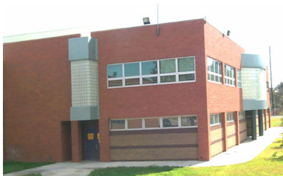
Figure E-46 Modern reinforced brick masonry.
