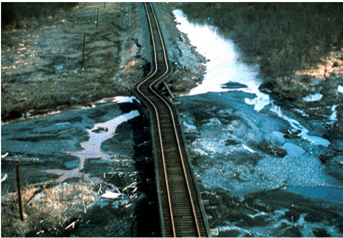
Transportation systems like railroads are fragile because a break in any spot can affect all traffic on the line. Ground response of loose, water-filled soils buckled this railroad bridge in the 1964 Alaska earthquake. Photo: USGS
