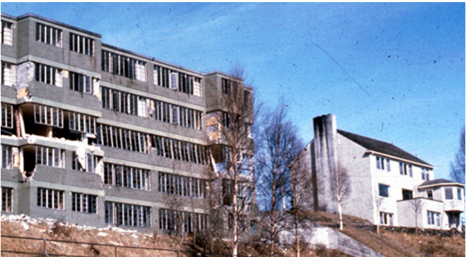
The interaction of building type and ground response can be seen in how these two buildings were affected by the 1964 Alaska quake. The Hillside Apartment Building had extensive damage, while the adjacent three-story wood-frame dwelling with the tall chimney had almost none. In general, when wood frame buildings in Anchorage were damaged, it was from some type of ground failure. Photo: USGS
