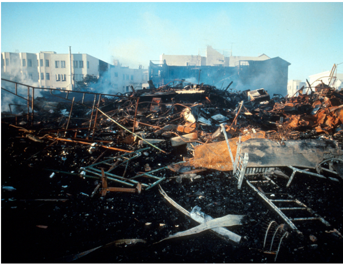
The ground response to earthquake waves can result in ruptured gas mains, which can start fires, and broken water mains, which makes it hard to fight fires. These smoldering remains are from the 1989 Loma Prieta, California earthquake. Photo: J. K. Nakata, USGS
