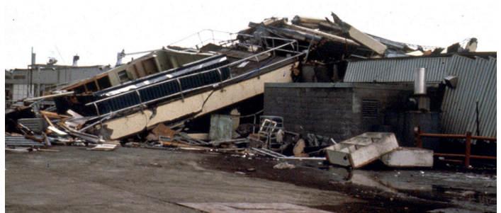
In 1964, the control tower at Anchorage, Alaska International Airport fell during the M9.2 earthquake. It was a split-level structure that was seven stories high on one side and built of reinforced concrete. Photo: USGS
