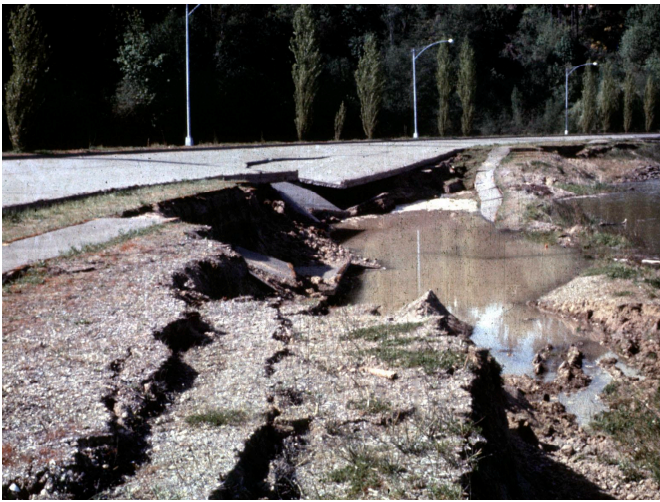
Liquefaction can destroy roads, as the 2001 Nisqually, Washington earthquake did to this street outside Olympia. Many stretches of Highway 101 and other coastal roads in Cascadia are vulnerable to this type of destruction. Photo: T. Walsh, Washington Division of Geology and Earth Resources
