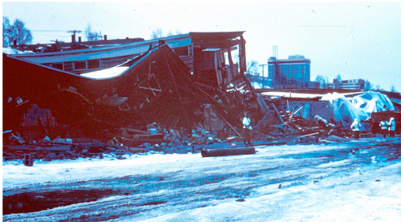
Warehouses at the toe of the Fourth Avenue landslide in Anchorage in 1964 were destroyed by compressional buckling and foreshortening. Much of the supply of food and drink for the city was stored in these buildings. Photo: USGS
