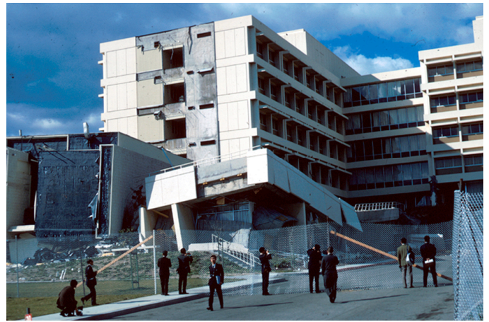
In the 1971 San Fernando earthquake, the south stair tower (above) fell, and there was other structural damage at Olive View Hospital. Three people died and the building was evacuated. It is imperative to have hospitals and other essential facilities available during the crisis of a subduction zone earthquake. Photo: R. Kachadoorian, USGS
