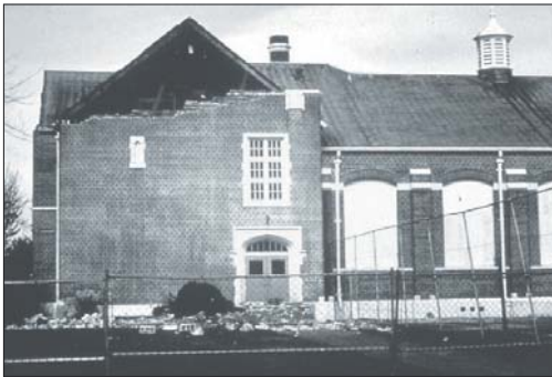
Structural Damage, Molalla High School, 1993 Photo provided by: DOGAMI
