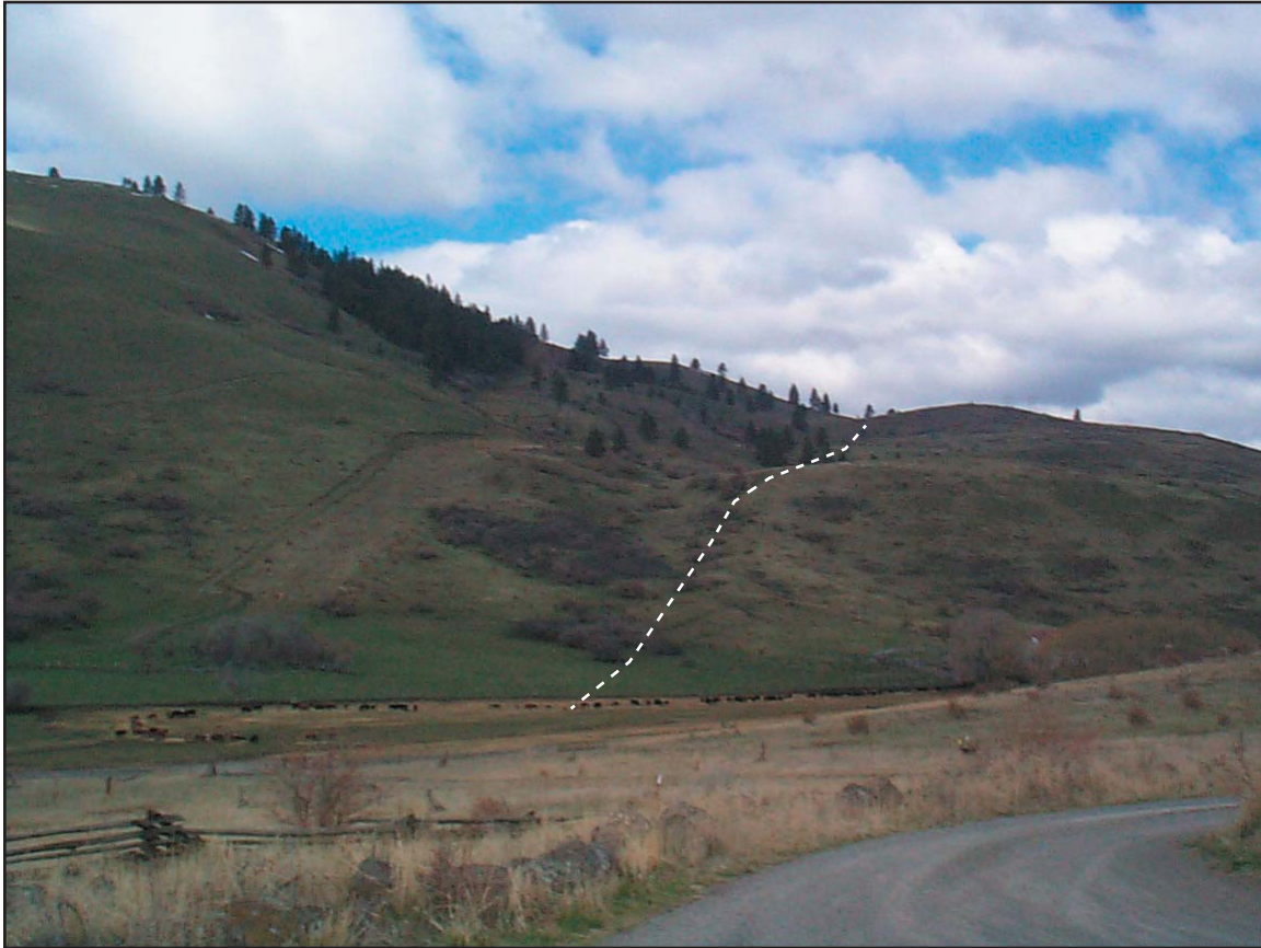
Figure 4. View to the west of the pipeline corridor that runs through a large landslide and debris flow complex. This is the route for natural gas, telephone, and fiber optic lines. The landslide buries the southern trace of what appears to be one of the more active faults in the area (dashed line).
