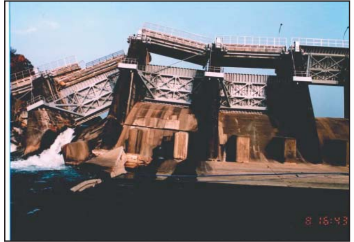
Figure 3.2. Failure of Shigang Dam in the 1999 Chichi Taiwan earthquake (Okunishi, K.).
