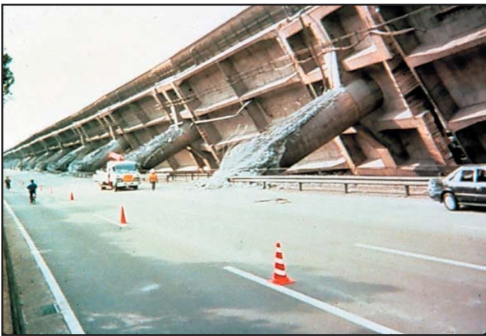
Figure 3.1. The Hanshin Expressway collapse in the 1995 Kobe, Japan earthquake (photo credit: Paul Sommerville).
