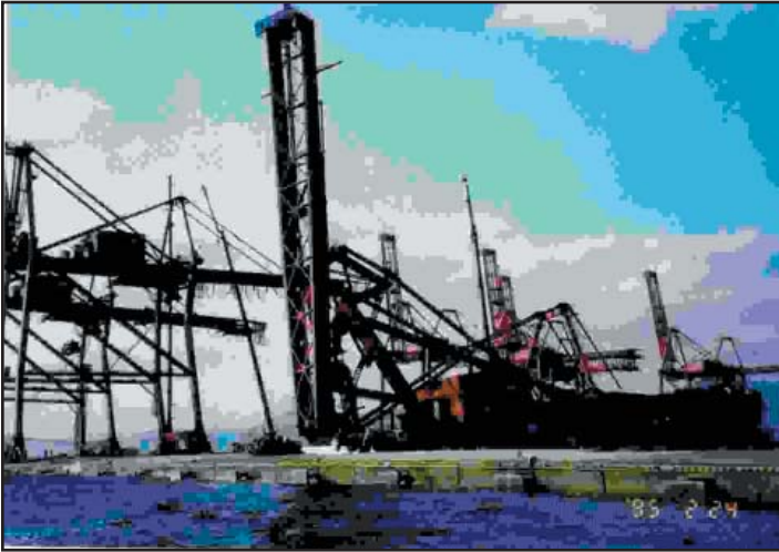
Figure 3.4. Failure of the port gantry cranes caused by liquefaction and lateral spreading during the 1995 earthquake at Kobe, Japan (photo: Ian Austin).
