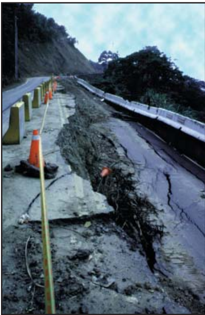
Figure 3.7. Outside edge of roads, which include fill material, commonly fail and limit the traffic flow to fewer lanes (Photo credit: David K Keefer).
