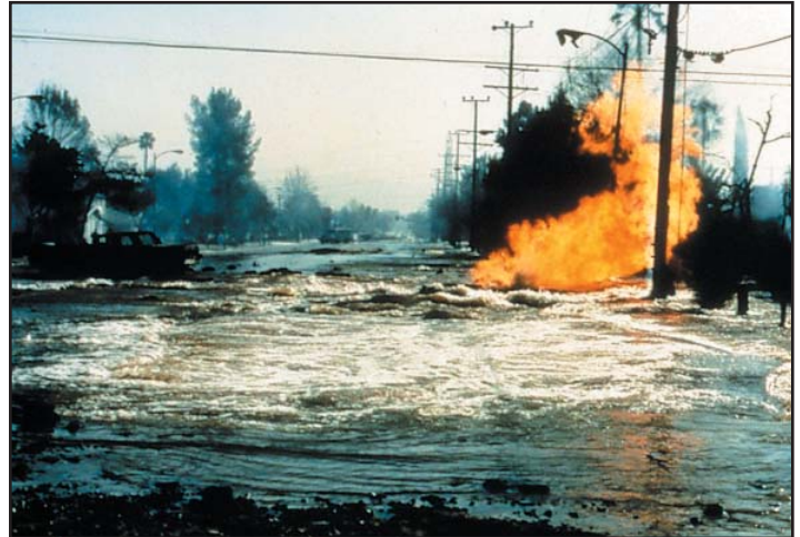
Figure 3.5. Co-located water and gas pipelines that failed in a California quake.
