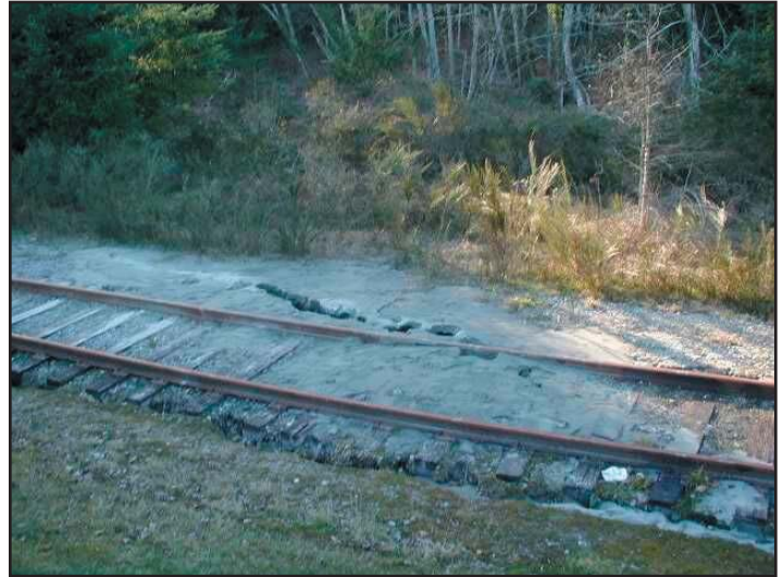
Figure 3.3. Damage to railway from liquefaction in the 2001 Nisqually, Washington earthquake (photo credit: William Byers).
