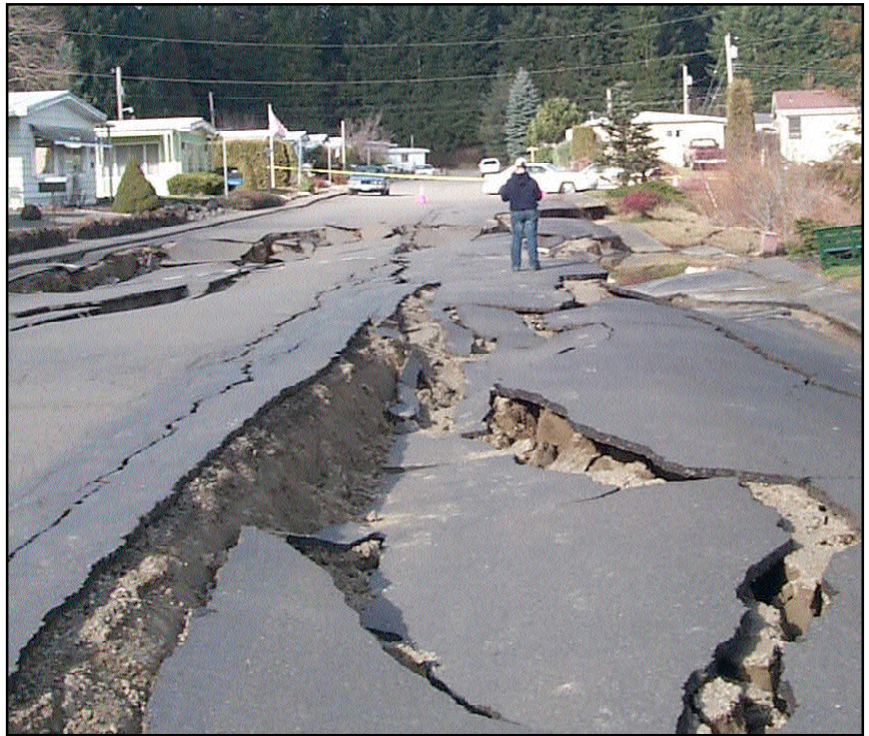
Figure 6. Liquefaction example from the 2001 magnitude 6.8 Nisqually earthquake.
