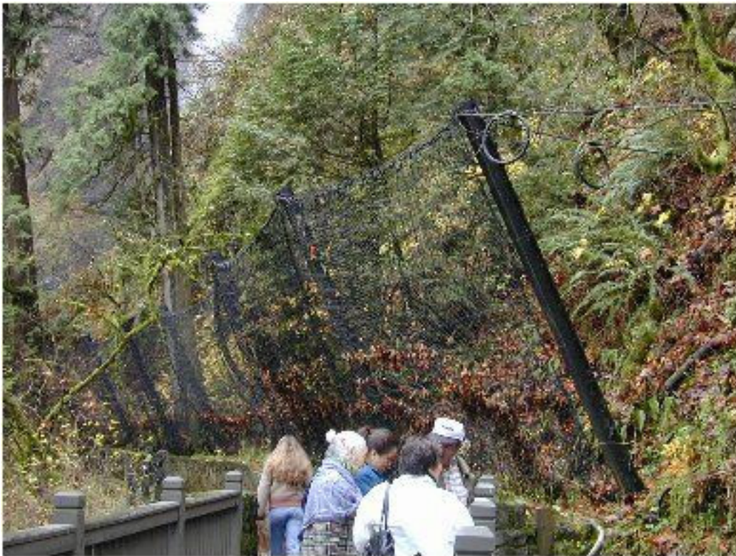
Figure 8. Multnomah Falls rock catchment net on footpath. This was installed by the USDA Forest Service as a result of a severe injury from a rockfall (modified from Wang and others, 2002)
