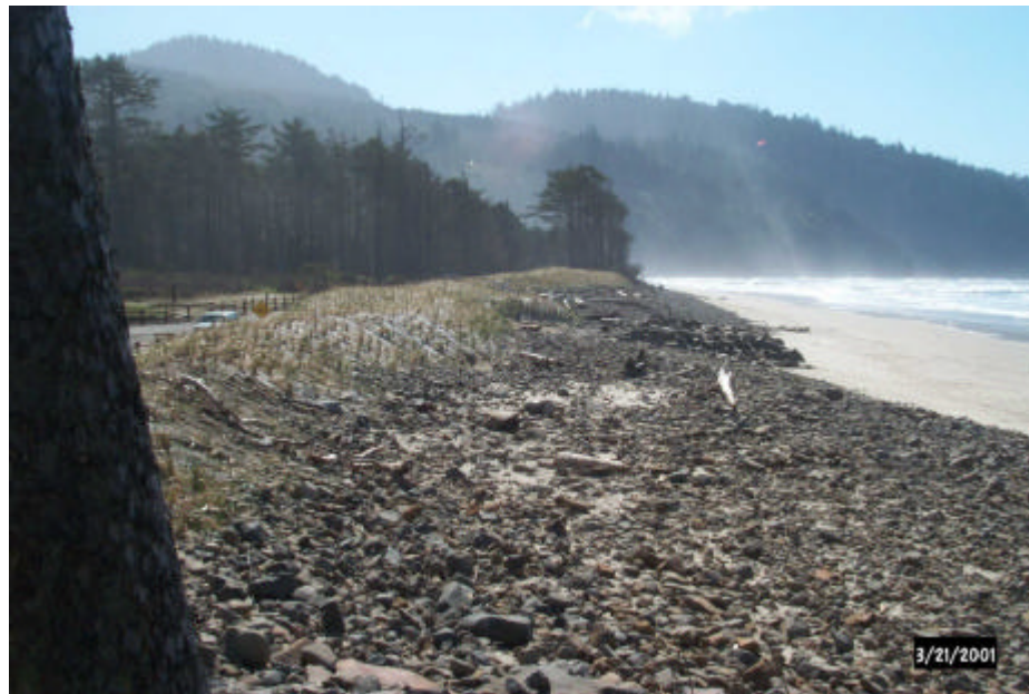
Figure 15 A dynamic revetment structure constructed at Cape Lookout State Park, utilizing materials found at the site.
