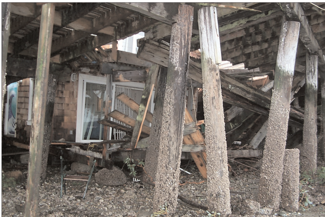
Photo 12. This home's collapse was caused by the Salmon Beach landslide – four houses were substantially affected as of 3-2-01.
