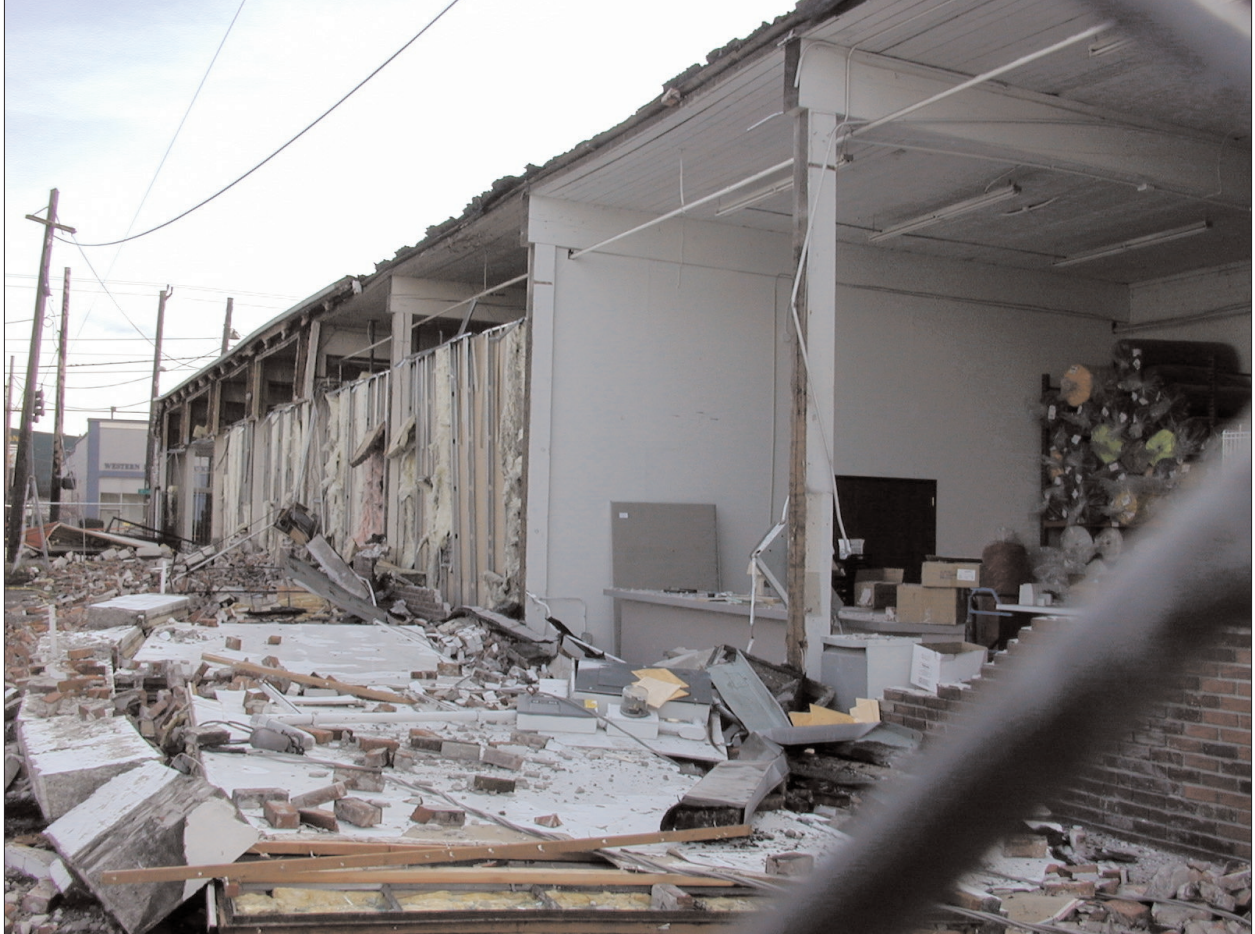
Photo 3. Failed concrete lintel above window bank not attached to girders in a URM building located near the intersection of S Forest St. and Utah Ave. S, Seattle.
