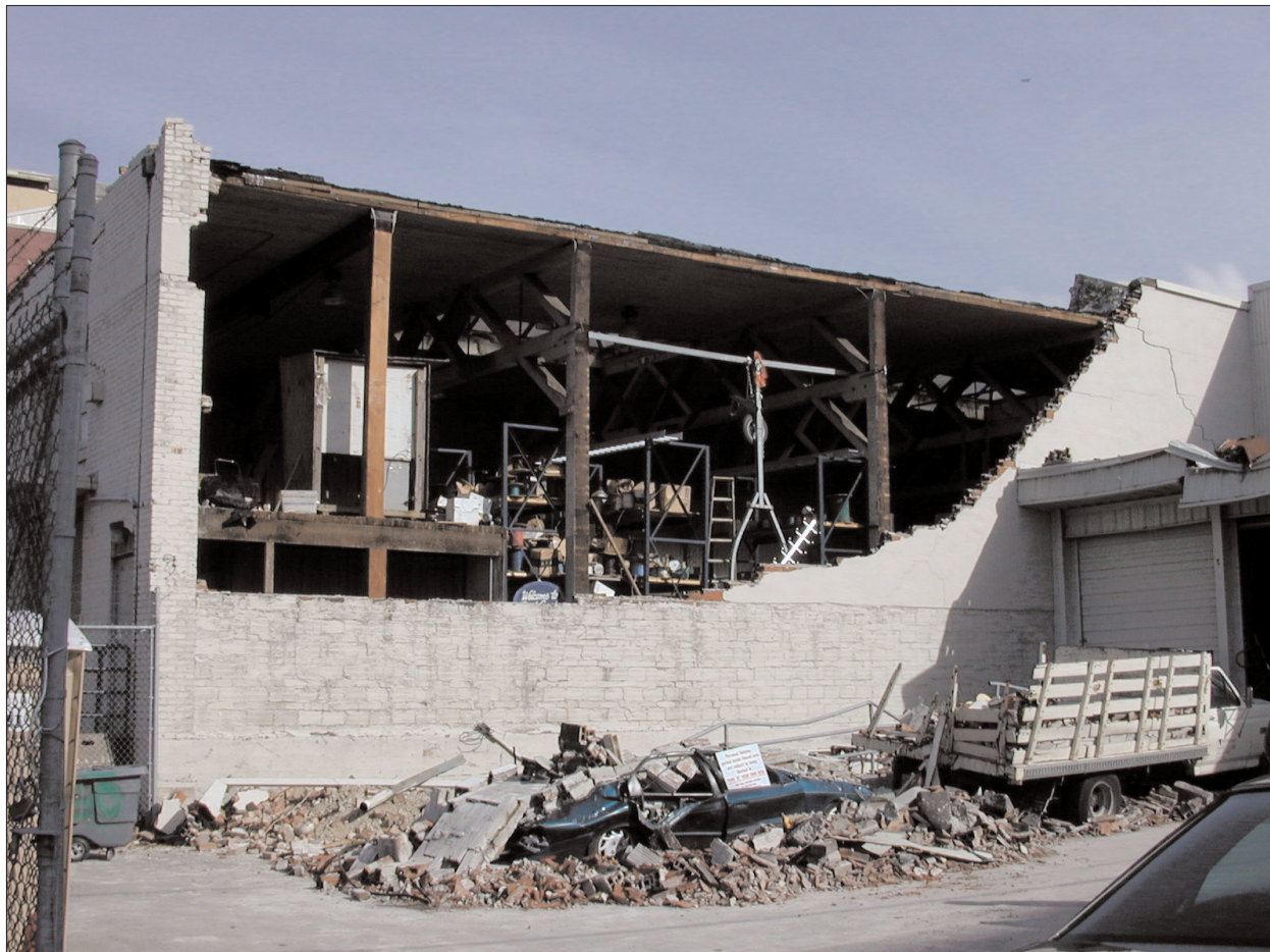
Photo 1. Collapsed hollow-clay tile wall at URM building located along Utah Ave. S in South Seattle.
