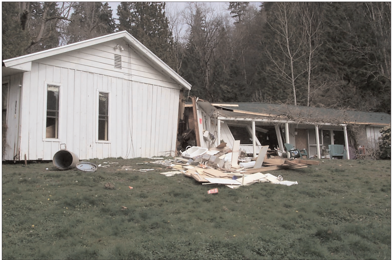
Photo 17. Damage at the Vanderossen residence in Maplewood from a debris flow that struck the back of the building seconds after the onset of shaking.
