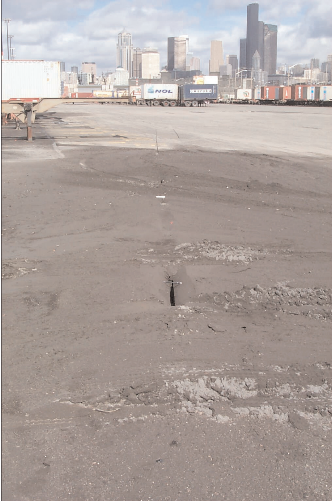
Photo 9. Sand boils from crack along utility trench in the Port of Seattle Terminal 30 – Seattle skyline in background.
