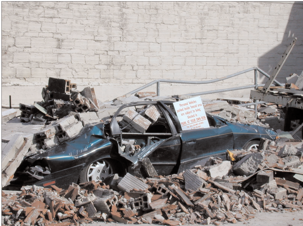
Photo 2. Close-up of a car crushed by the failed wall – the same building on Utah Ave. S in Seattle.
