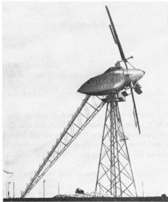
Figure 2. Aerogenerator of Russian design built at Yalta near the Black Sea in 1931.
