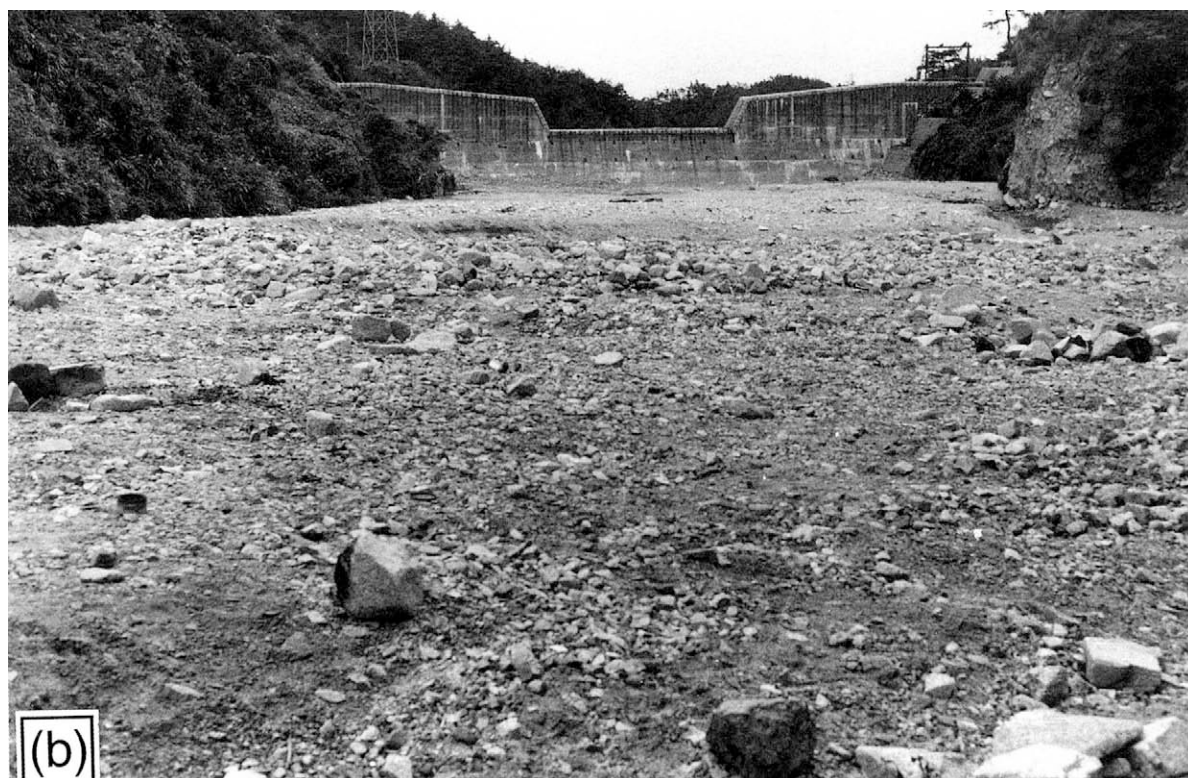
Figure 33. Check dam in Hyogo, Japan (30 m high, 78 m long, storage capacity 300,000 m 3 ), (a) before and (b) after a debris flow. (Photo from United Nations, 1996)
