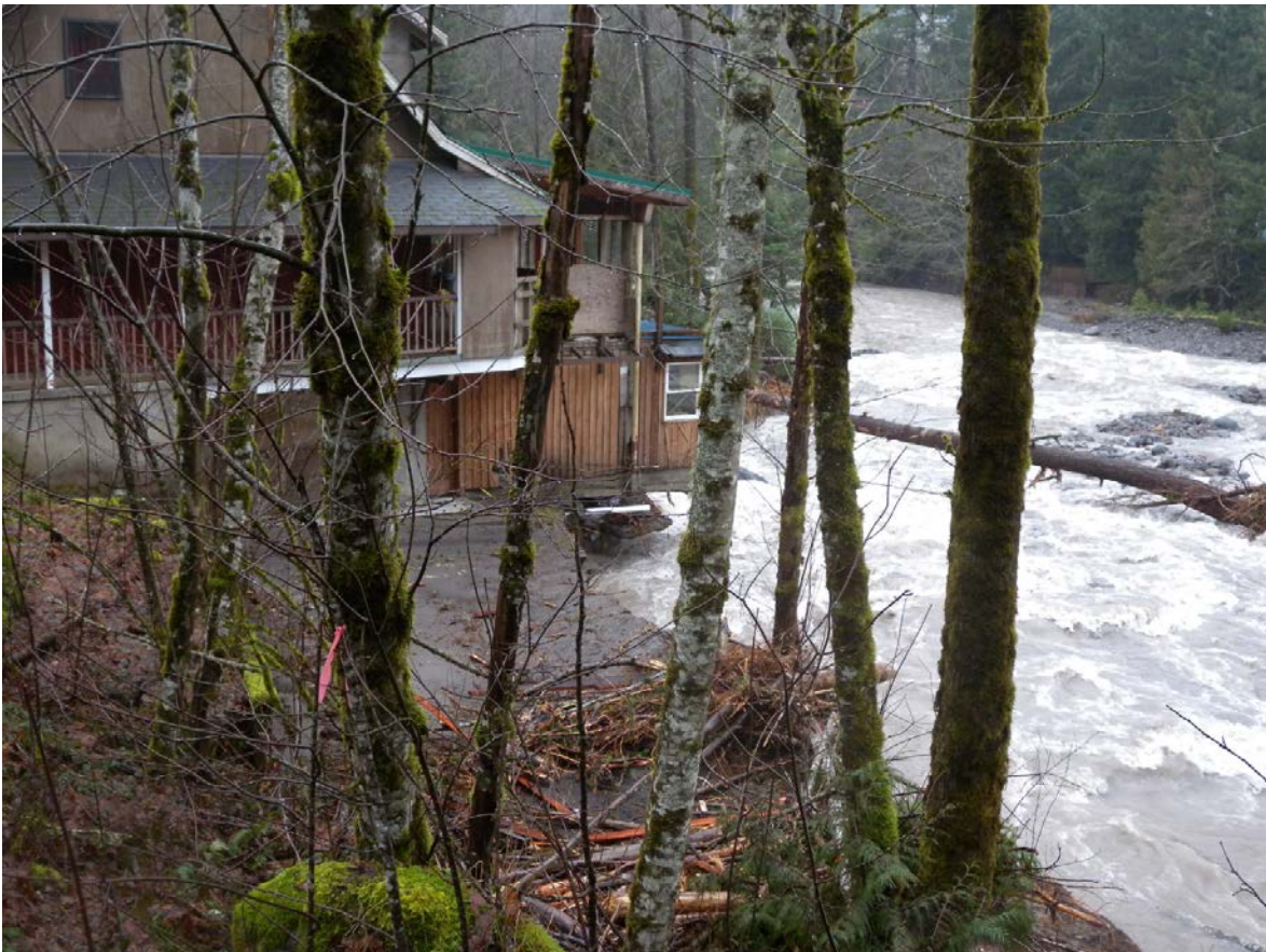
Figure 2-1. Private residence undercut during a flood and channel migration event in January 2011 on the upper Sandy River in Clackamas County, Oregon (photo credit: J. English, DOGAMI, 2011).
