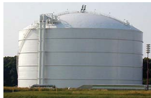
LNG storage tanks are built like huge insulated bottles to keep the gas liquefied and at a very low temperature.
