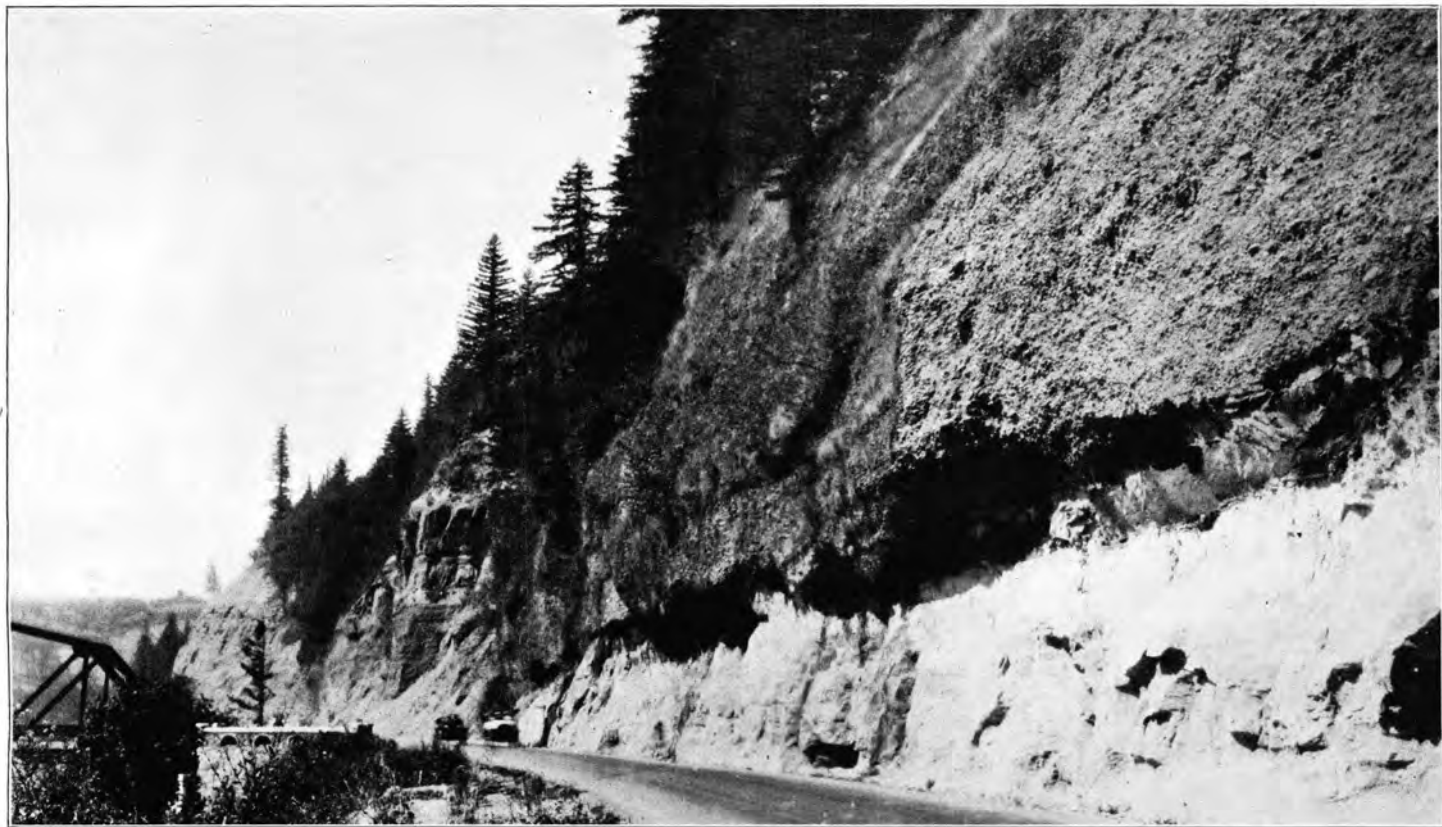
Cornice of coarse cemented gravel overhanging less resistant sandstone. Auto Club bridge and Columbia River Highway
