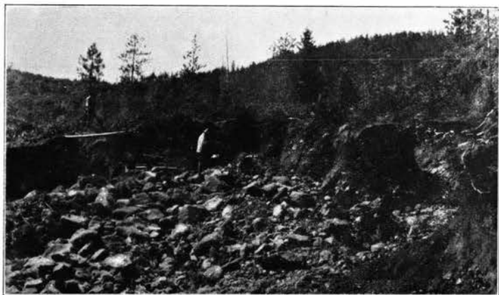
Fig. 36. Pit produced by ground sluicing on Mark Wood's prospect near Spokane creek
