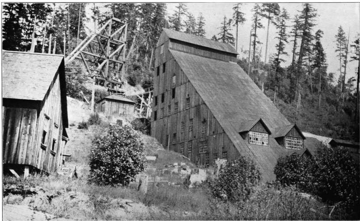
Plate IX. 20-stamp mill and hoist at the Granite Hill mine near Grants Pass, Oregon.
