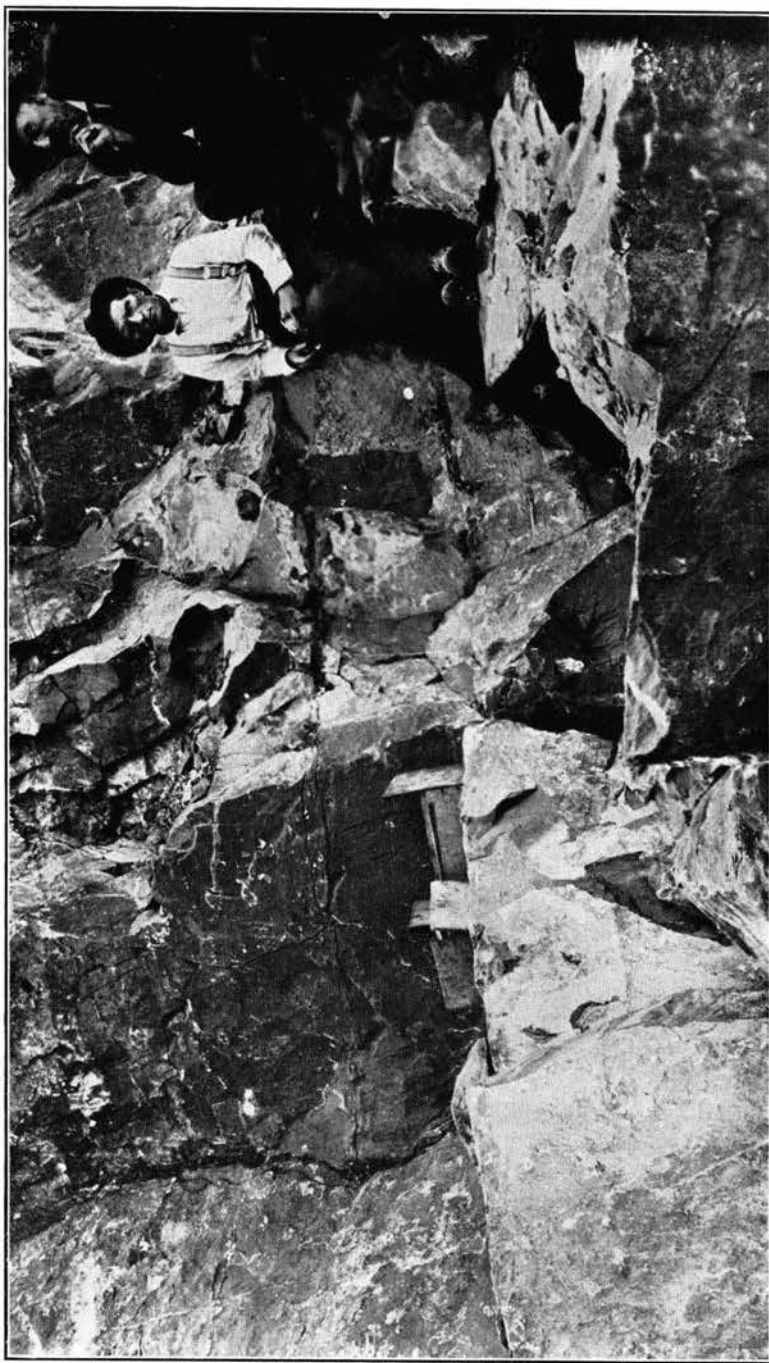
Black Marble Quarry, Wallowa County, showing jointing and size of blocks.
