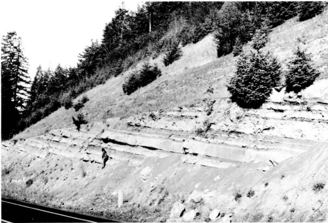
Figure 4. Rhythmically bedded sandstone and siltstone of the Tyee Formation of middle Eocene age. Road-cut exposure along State Route 20, 4 miles east of Toledo, Oregon (Stop 1).
